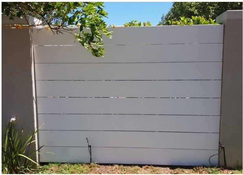
Nutec "Handi-planks" fibre cement closers (with visible gaps for increased visual permeability)
