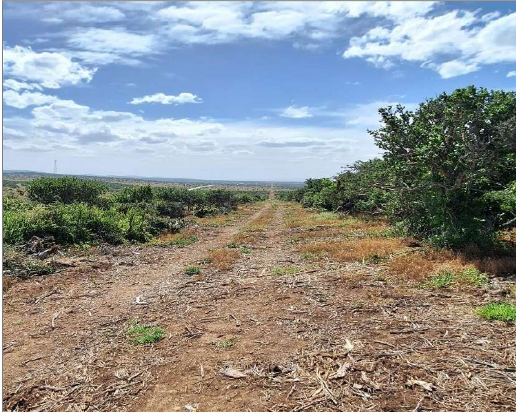
Figure 3: Access Road established for OHPL
