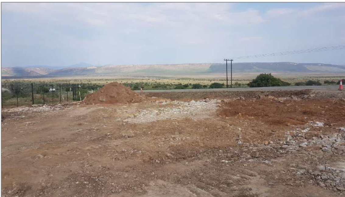
Figure 5: Widening of main access point for WEF at R75.
