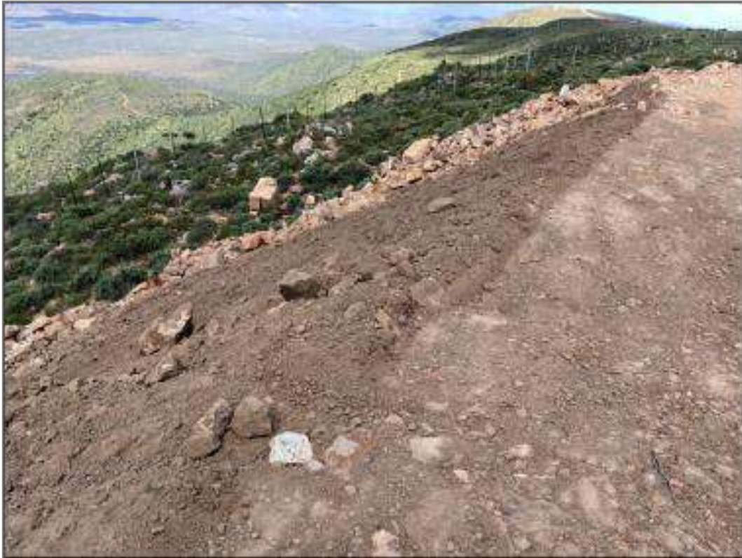
Figure 8: Topsoil being placed on slopes for rehabilitation.
