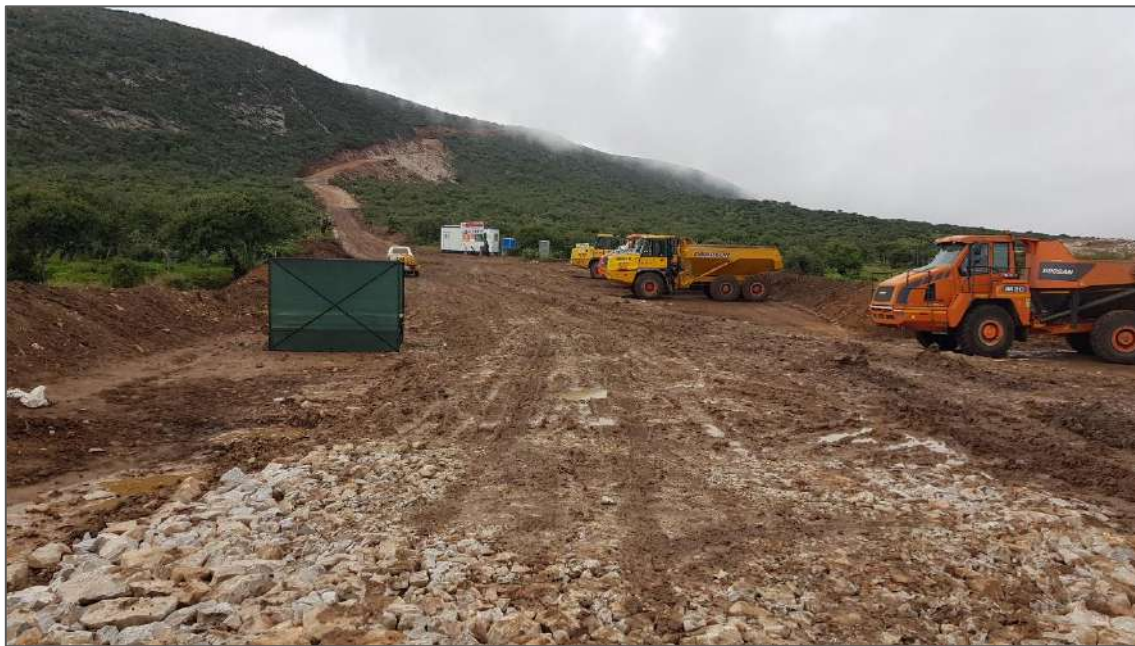
Figure 4: Measure being implemented to assist in drainage at the laydown area.
