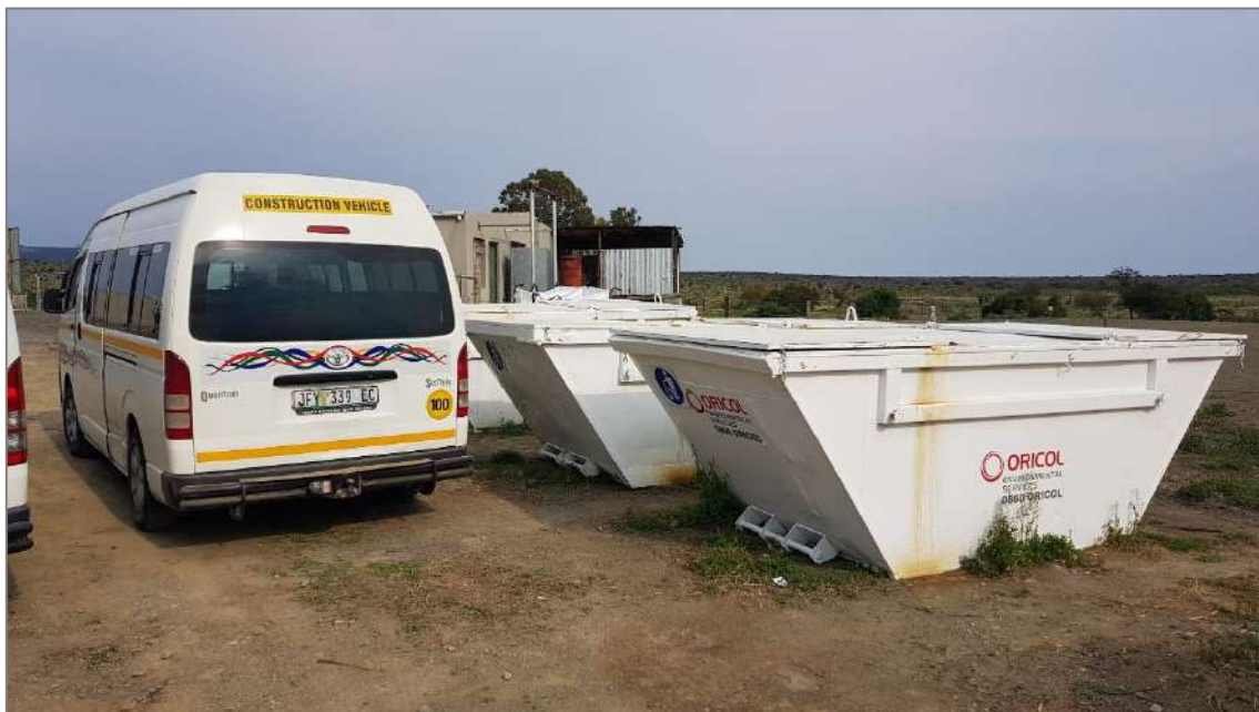
Figure 2: Access to waste skip impeded.
