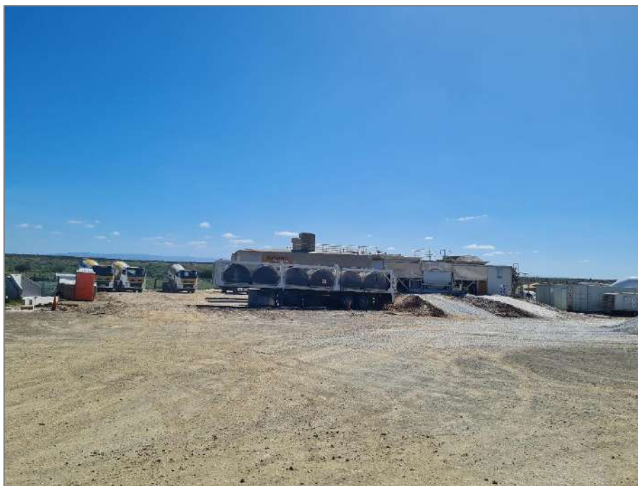
Figure 5: Operational mobile batch plant
