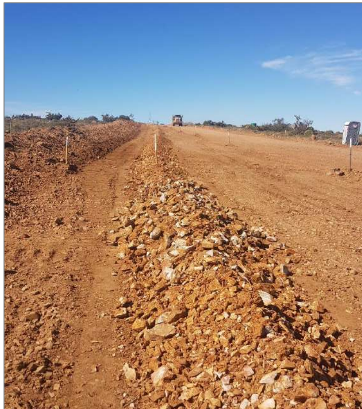
Figure 4: V Drain installed for water run off management.
