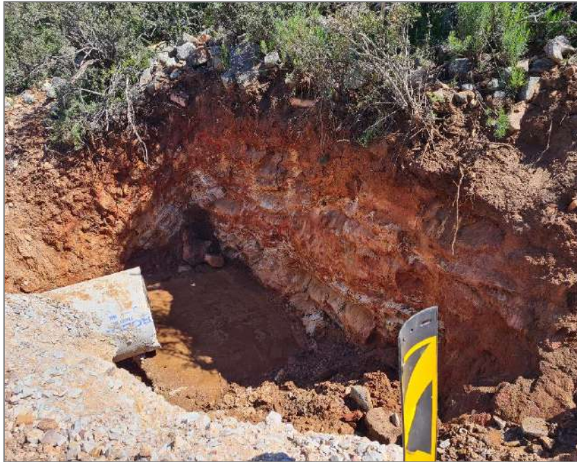
Figure 3: Culvert installation on the main access route.
