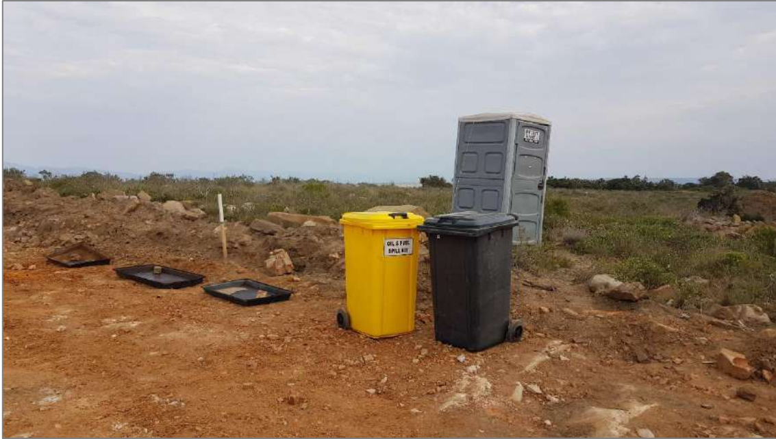
Figure 3: Spill kit and drip trays on site.
