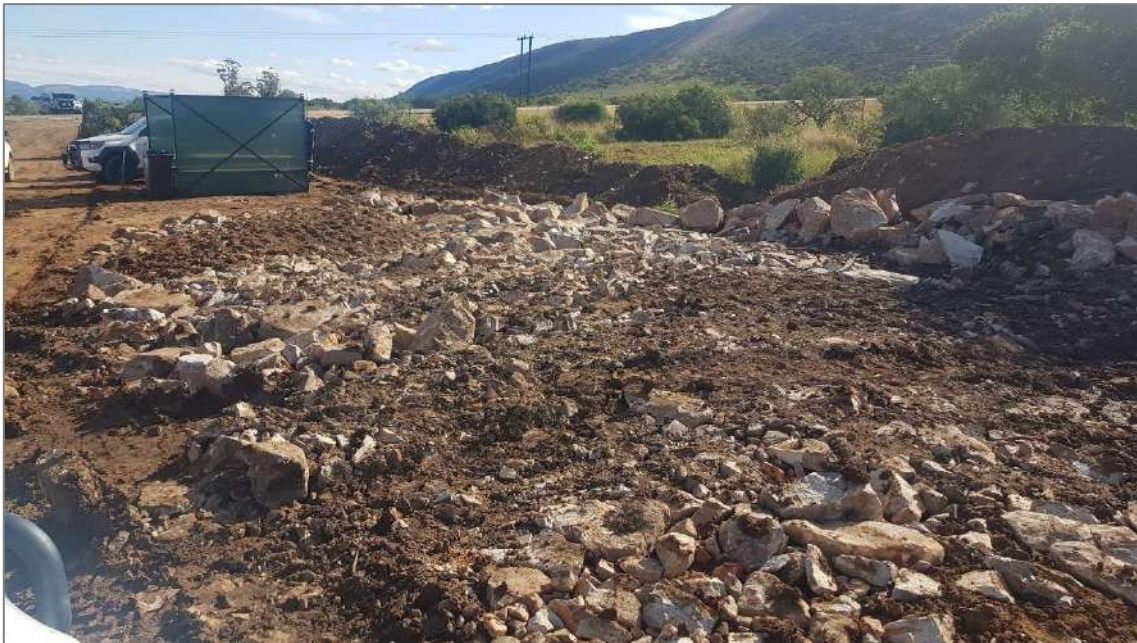
Figure 2: Measure being implemented to assist in drainage at the laydown area.
