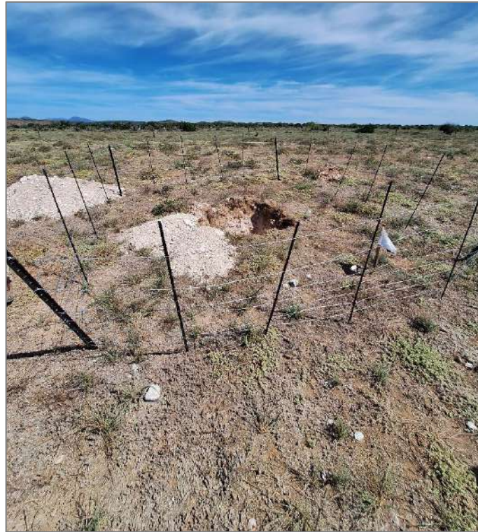
Figure 4: Barricading located round OHPL excavations.
