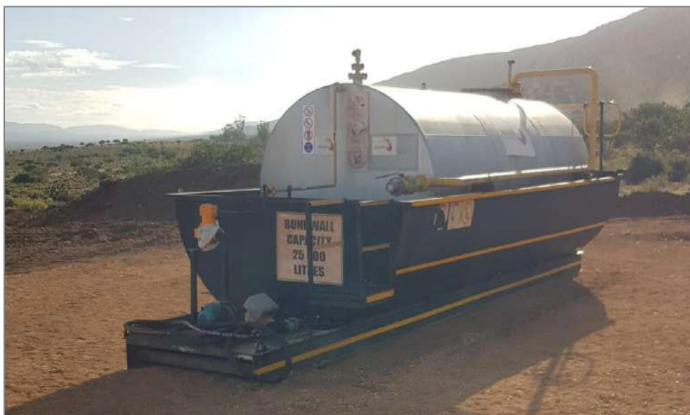
Figure 3: Bulk fuel storage container which arrived on site. Was not in use at the time of site visit.
