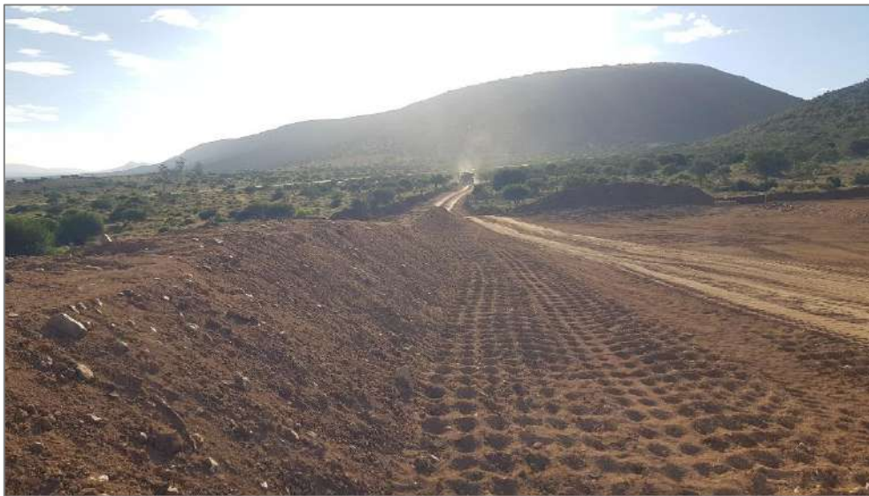
Figure 5: Topsoil be neatly stored at the laydown area.
