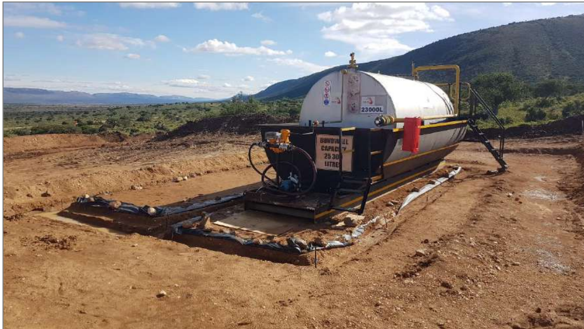
Figure 3: Works commencing on bunding for bulkf fuel storage container.
