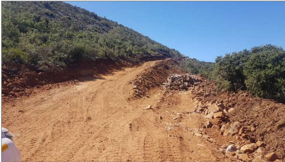
Figure 5: Start of main access route to turbine positions.
