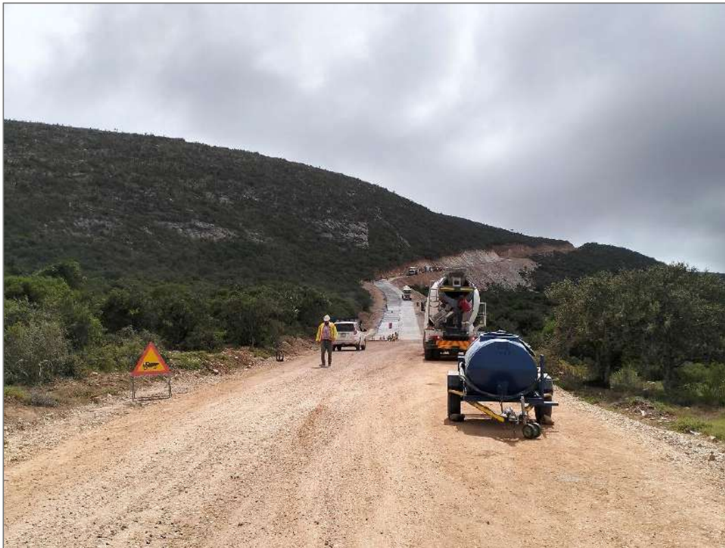
Figure 6: Concrete on the Main access road.
