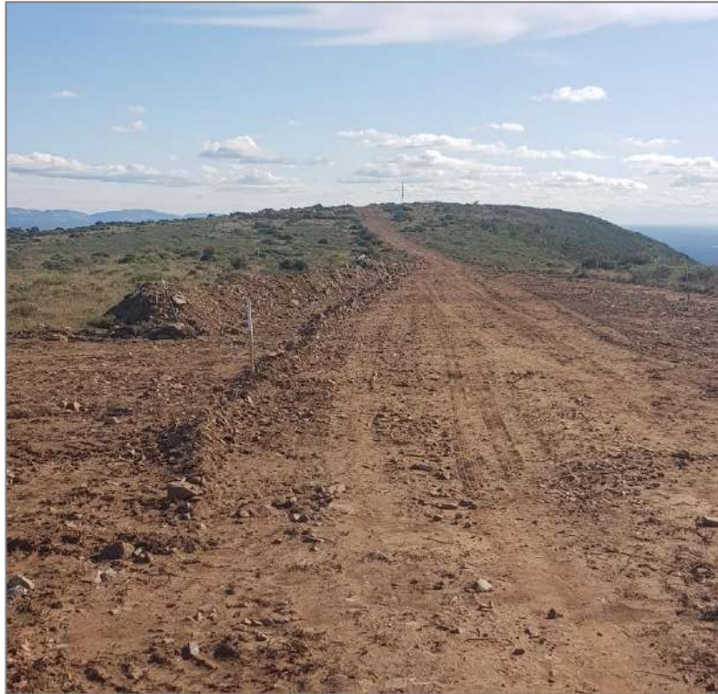
Figure 4: View of internal access road as seen from turbine position.
