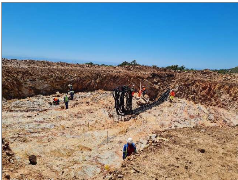
Figure 4: Cleaning of base excavations
