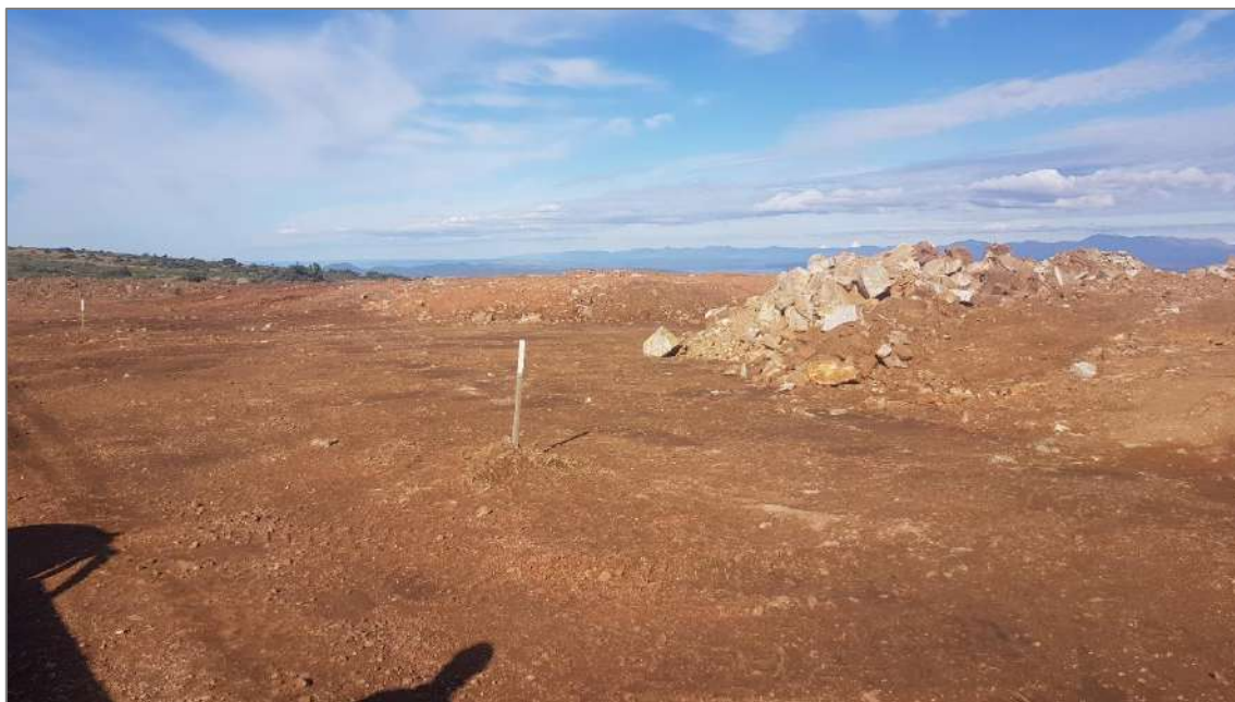
Figure 5: Stockpile of material for access route. Stockpile is well maintained.
