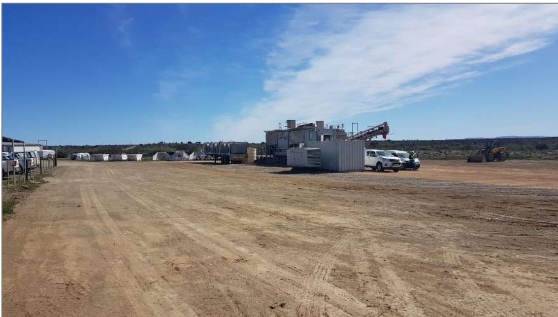
Figure 5: Mobile batch plant
