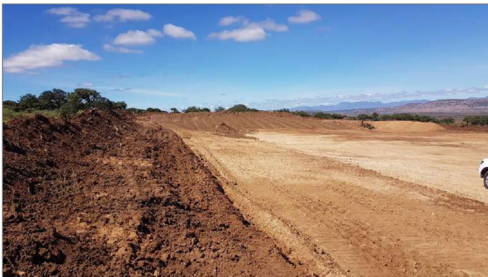
Figure 4: Topsoil being stored along the perimeter of the site laydown area.
