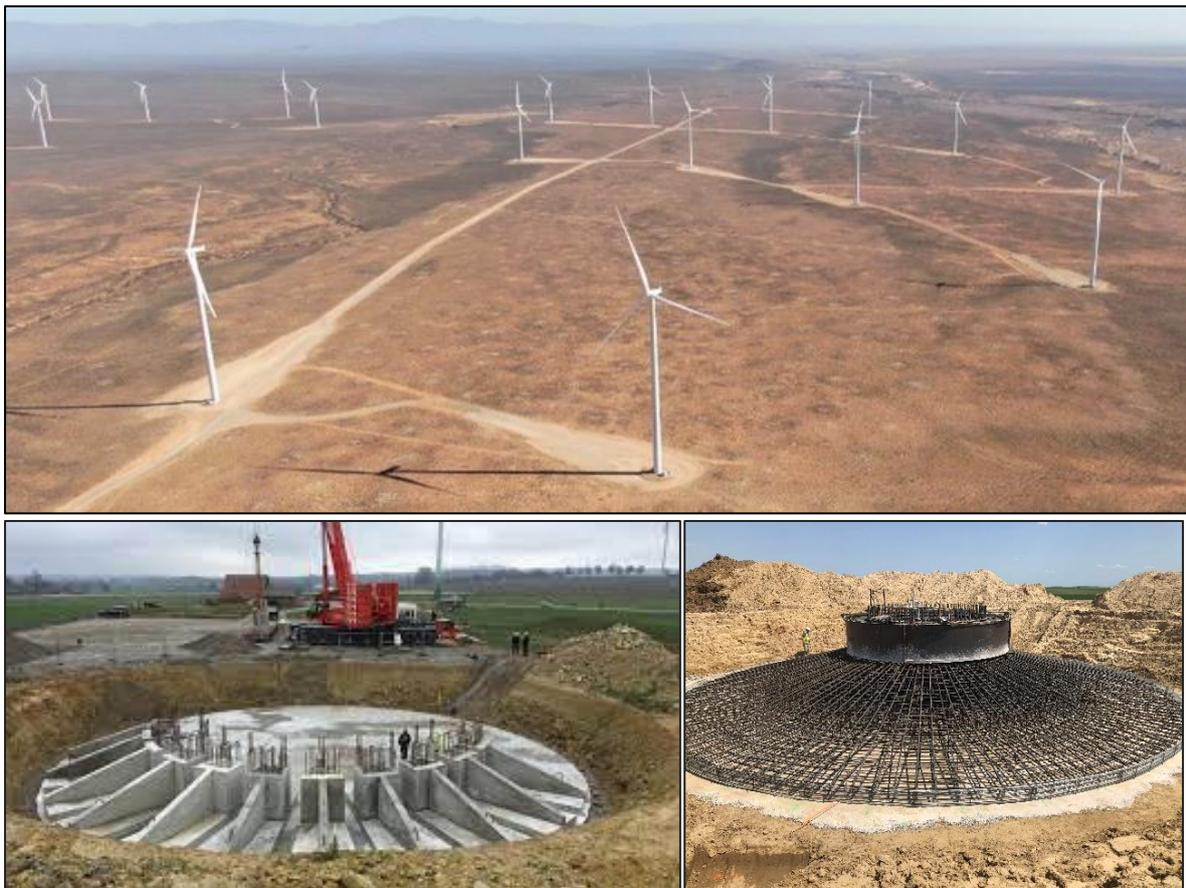
Figure 6-1 | Typical installation and foundation examples for the WEF including the crane pad
