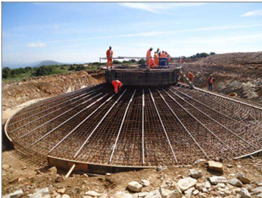
Figure 1: Preparation for concrete pouring at base foundations.
