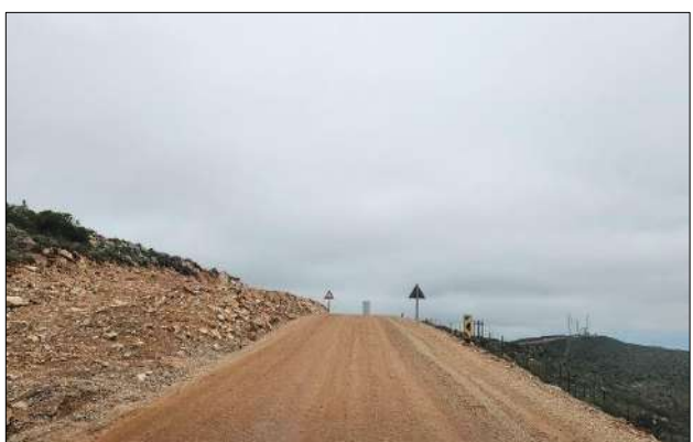
Photo 3b: Sloped gravel road section, no erosion observed.
