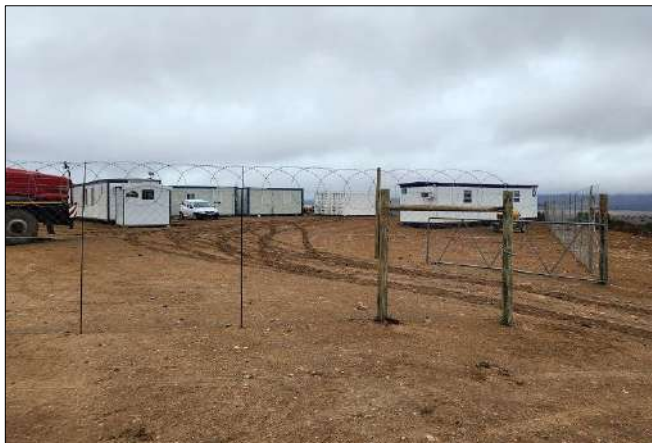
Photo 7c: Vestas offices established since the previous audit.
