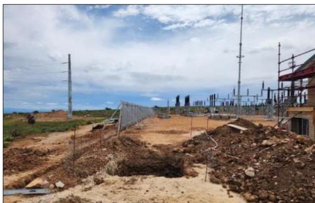
Photo 8a: Construction of steel fencing around substation.
