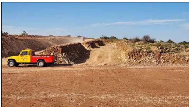
Photo 7a: Earthwork preparations for turbine components.
