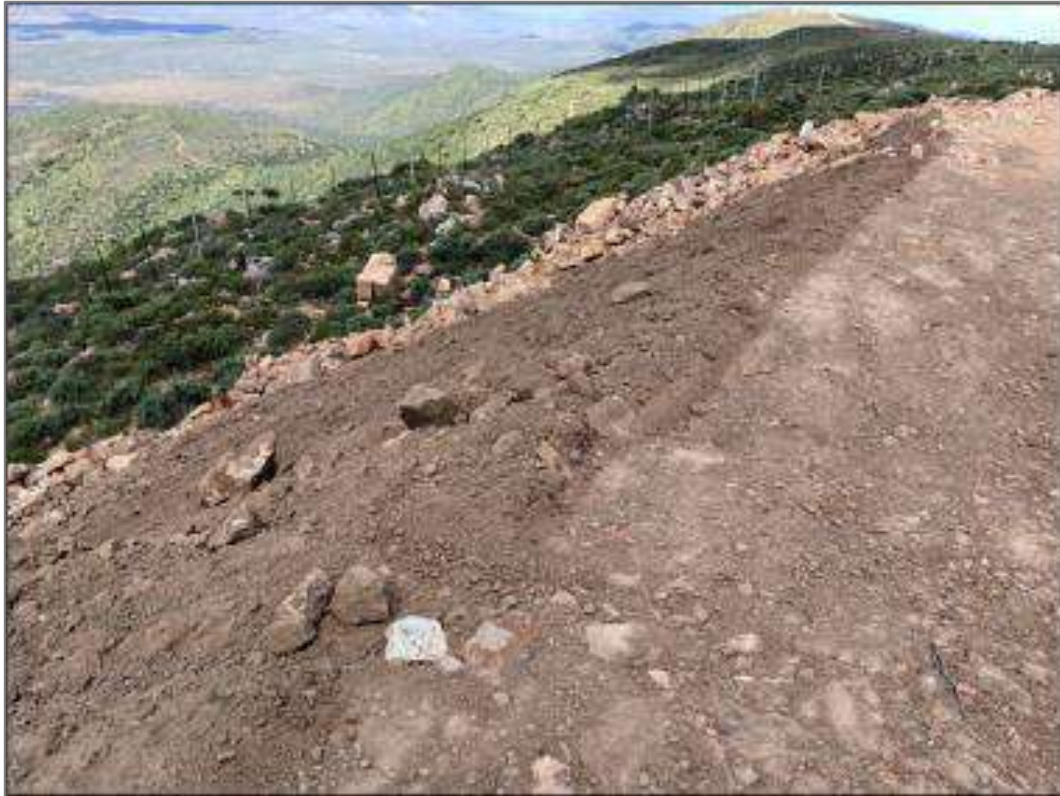
Figure 8: Topsoil being placed on slopes for rehabilitation.
