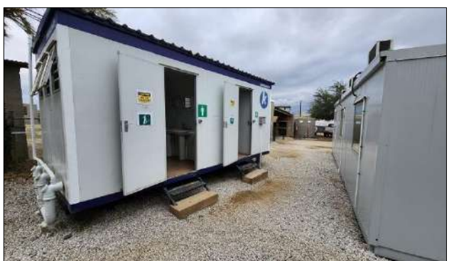
Photo 7b: Temporary ablutions connected to conservancy tanks which are serviced as and when required.
