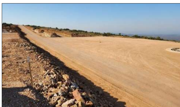
Photo 2a: Levelled and compacted turbine hardstand.
