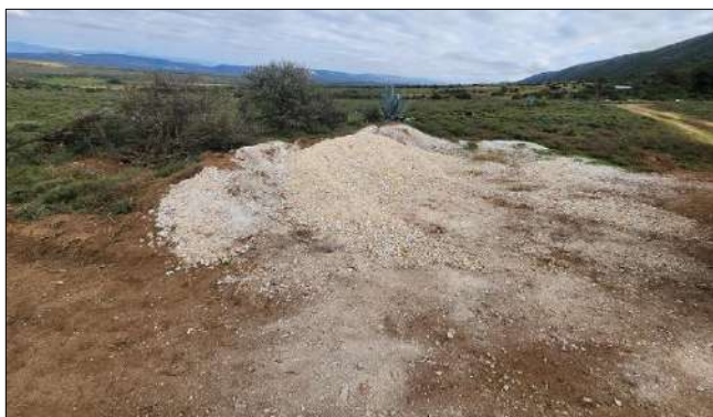
Photo 5c: Imported G5 material for backfilling the stay foundations.
