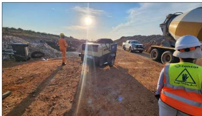
Photo 2a: Drip tray observed under a mobile generator.
