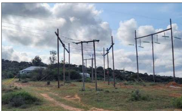
Photo 5d: Timber supports in place to protect existing line before stringing commences.
