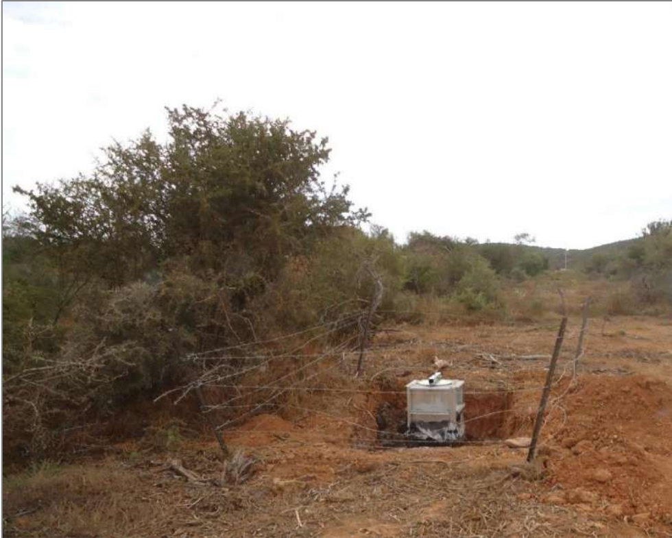
Figure 4: Barricading of open excavations on OHPL works.
