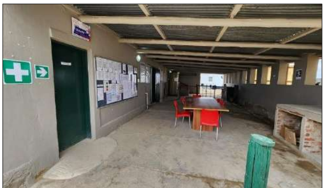
Photo 5b: Good housekeeping at the site office.
