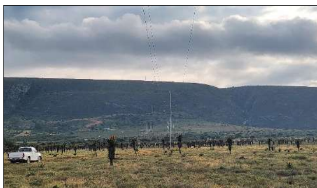
Photo 4c: Good state of vegetation along the servitude.
