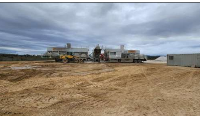
Photo 6b: Concrete batching facility.
