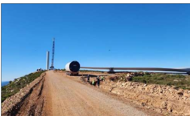
Photo 4a: Erection of one of the wind turbines underway.
