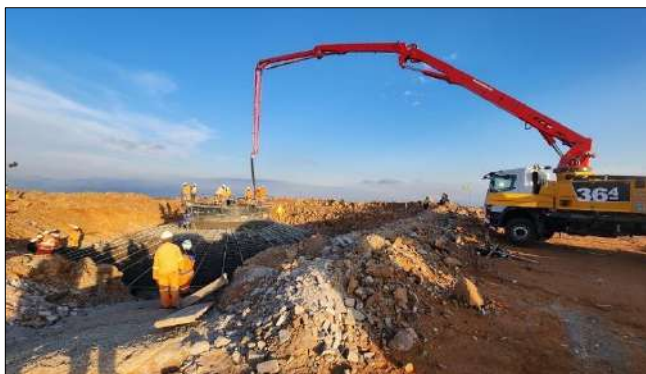
Photo 1a: Concrete pour underway at a turbine location.
