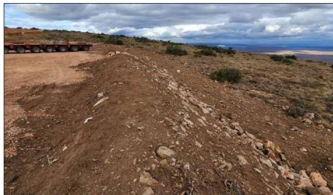
Photo 2a: Topsoil returned to sloped edges of hardstands.
