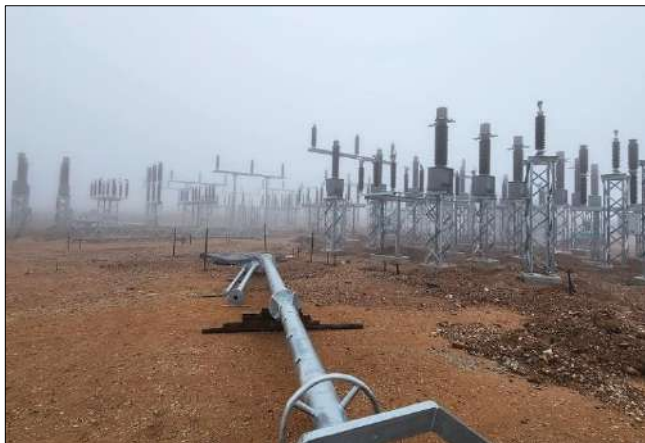
Photo 9a: Civil construction progress at the substation.
