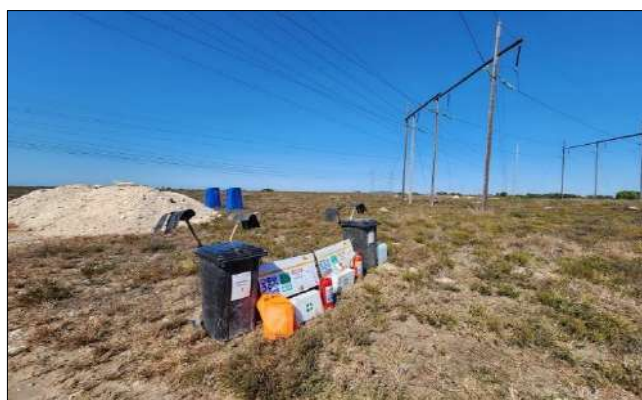
Photo 2c: Ablution and protective measures at CR2 (bins, fire equipment, signage, drinking water).
