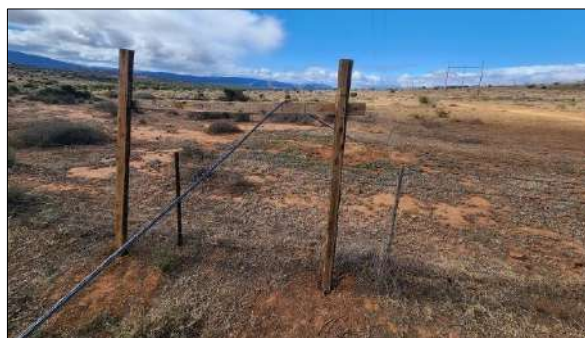
Photo 8c: Protection of farm fences observed during pulling of pilot cables.
