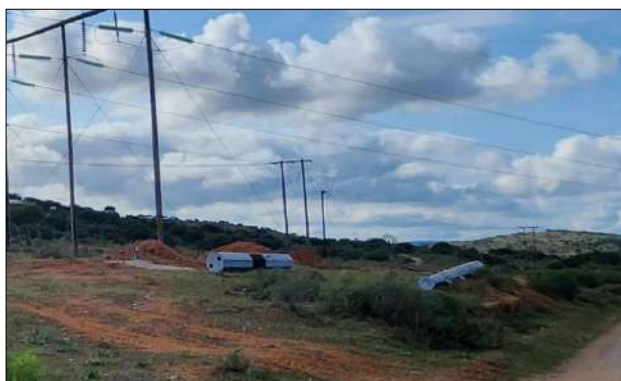
Photo 6d: Steel monopole components delivered to site prior to erection.
