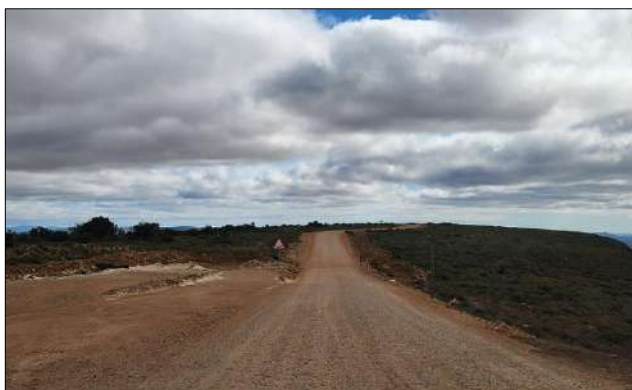
Photo 5b: Section of road with earthen stormwater drains.
