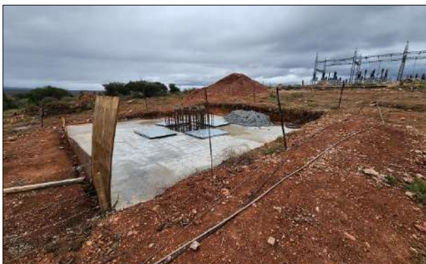
Photo 4d: Terminal tower foundation (WK3) outside Wolf SS.
