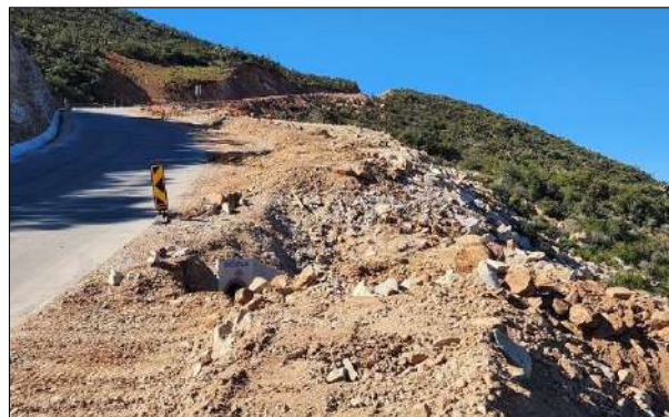
Photo 8b: View of the road's fill slope embankment.
