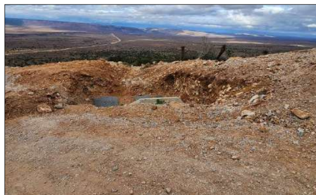
Photo 8b: Gabion and culvert installations underway.
