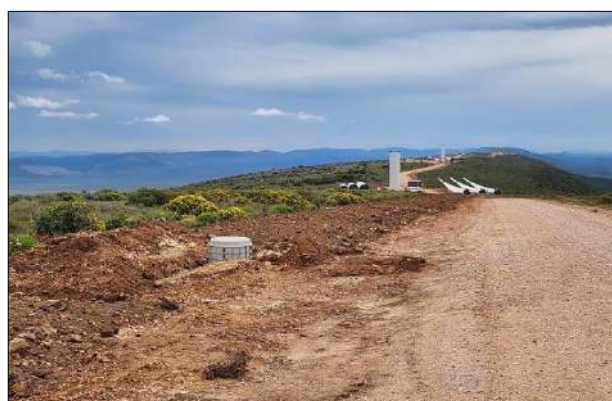
Photo 4b: Levelling/backfilling of cable trench in progress.
