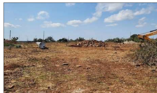
Photo 8c: Barricaded excavations at CR120.
