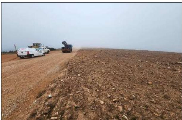
Photo 6b: Rehabilitated road siding/vehicle turning point.
