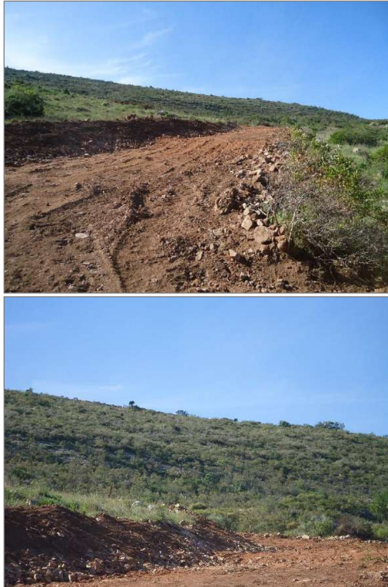
Figure 8: An existing farm road that was widened on the 13km OHPL.
