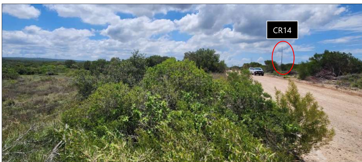
Photo 6d: NE view where seven tower positions were deviated beyond the 100m Grassridge-Skilpad powerline corridor (situated on the left side of the gravel road) on farm property Geluksdal No. 590.
