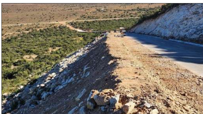
Photo 7b: View of fill slope (left) and cut/back slope (right).
