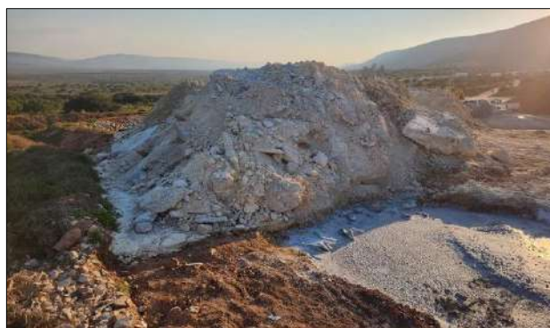
Photo 8a: Concrete spoil stockpile at the temporary laydown area.
