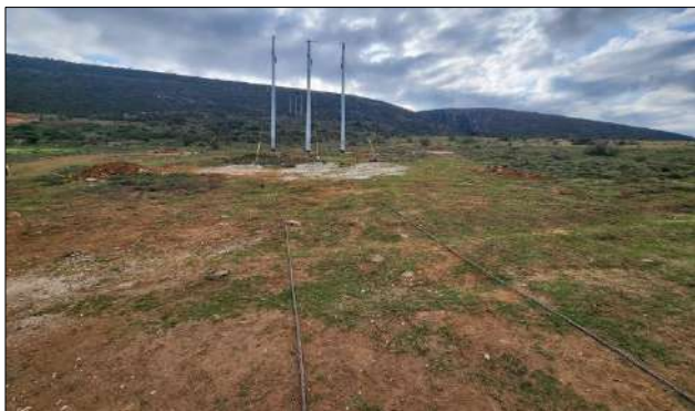
Photo 1c: & Photo 2c: Stringing of conductor cables aided with pilot cables observed to be underway.
