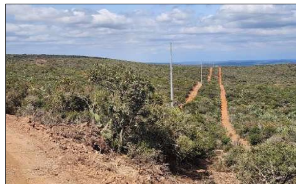
Photo 6c: Erected towers on the Dassies' Ridge property.
