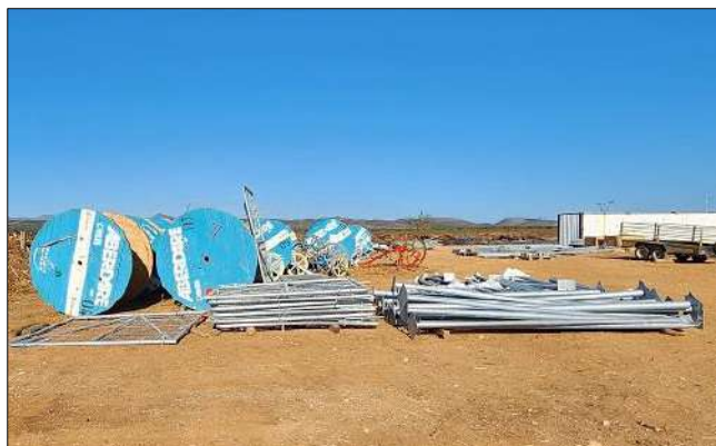
Photo 2b: Good housekeeping observed at the site camp.
