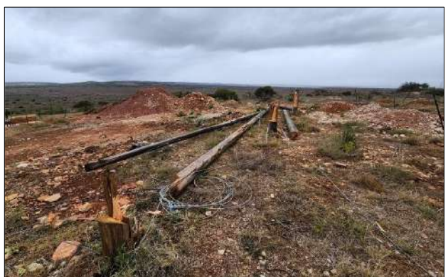
Photo 5d: Dismantlement of timber pylons is underway on the existing Wolf-Skilpad line.
