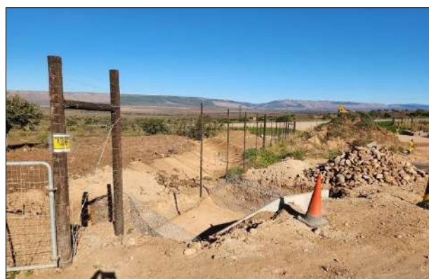
Photo 4b: Installation of gabions for stormwater run-off.
