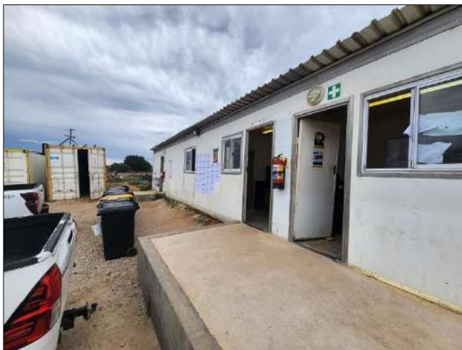
Photo 1c: Waste bins available at Wolwefontein laydown area.
