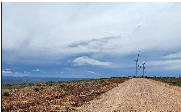
Photo 1b: Incomplete section of MVA cable trench.
