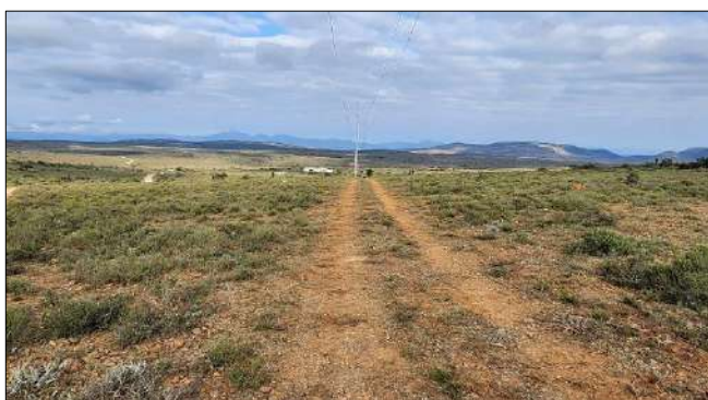
Photo 7c: General good condition of the farm access roads.
