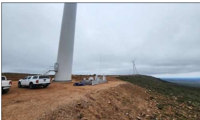
Photo 5a: Some germination of grass and forbs observed on the hardstand edges, no invasive vegetation observed.
