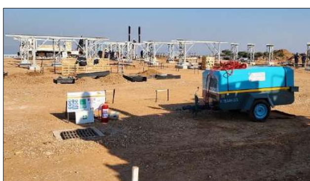
Photo 4a: Civil construction continues at the WEF substation.
