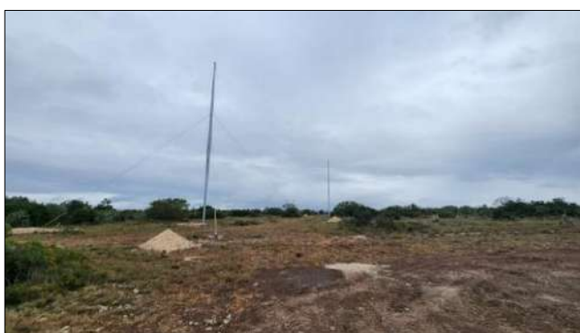
Photo 3d: View north of towers erected near Grassridge SS.
