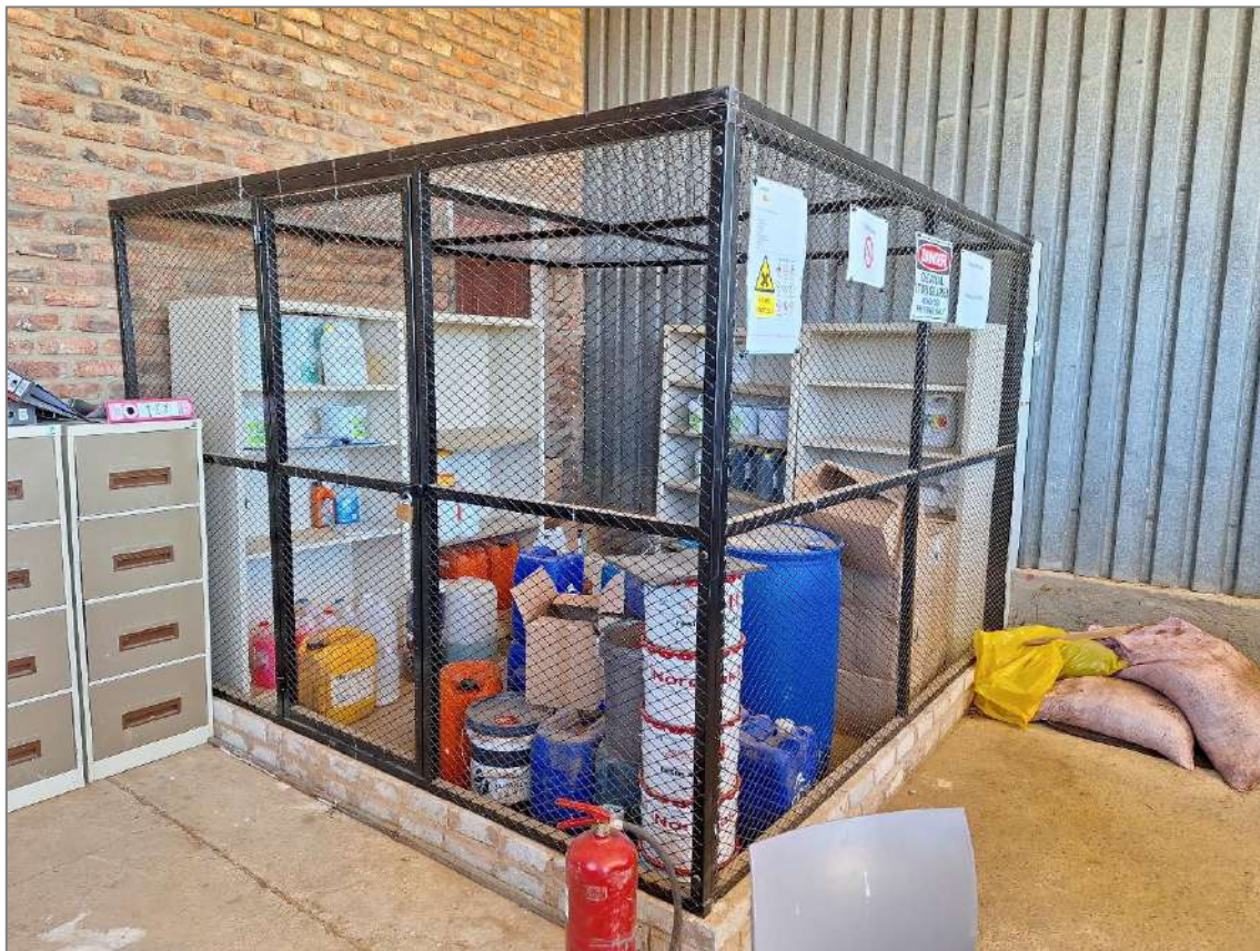
Figure 3: Hazardous store container located at site offices.
