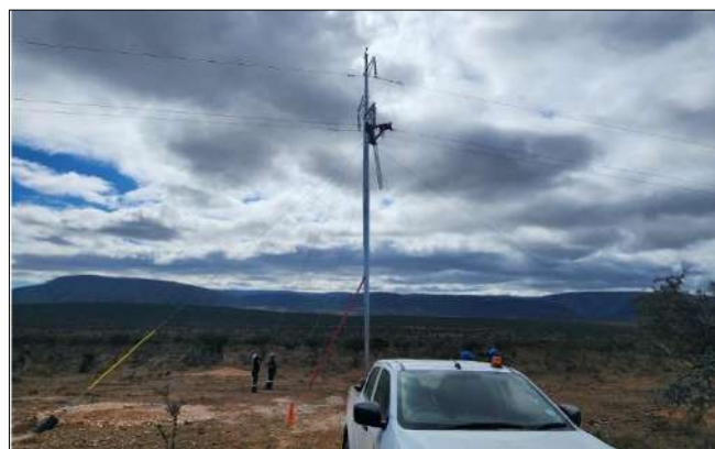
Photo 6c: Clamping of insulators underway on the SW line.
