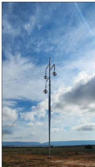
Photo 1c & Photo 2c: Preparation for stringing of conductor cables using pilot cables observed underway.
