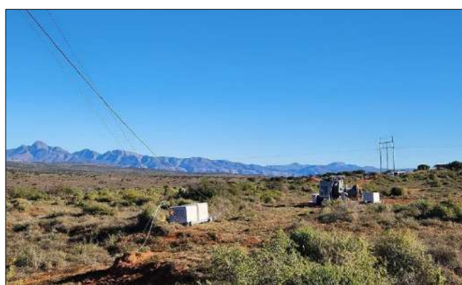
Photo 4c: Back-stayed tower WK5. Pulling of pilot cable underway.
