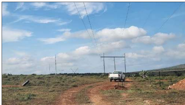
Photo 2d: New steel monopoles adjacent to the existing line.
