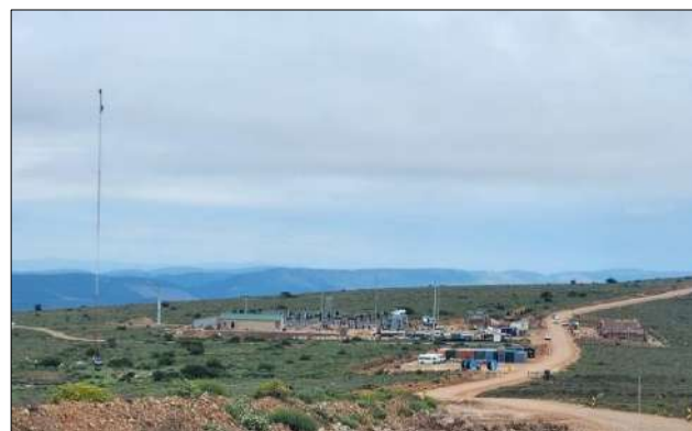
Photo 6a: View of civil construction progress at substation.
