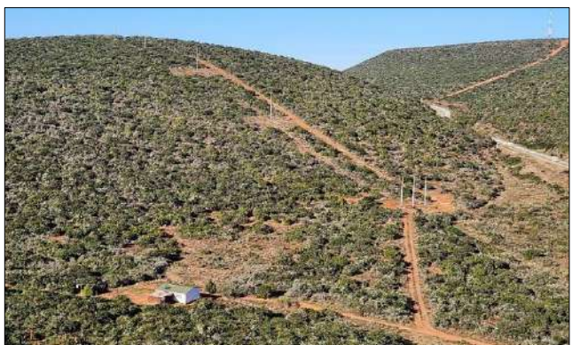
Photo 5d: Access between CR152 & CR147, still to be strung.
