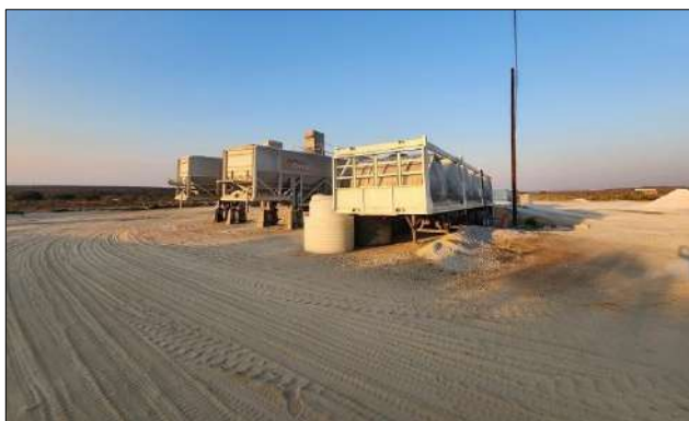
Photo 5b: Demobilising of concrete batch plant underway.
