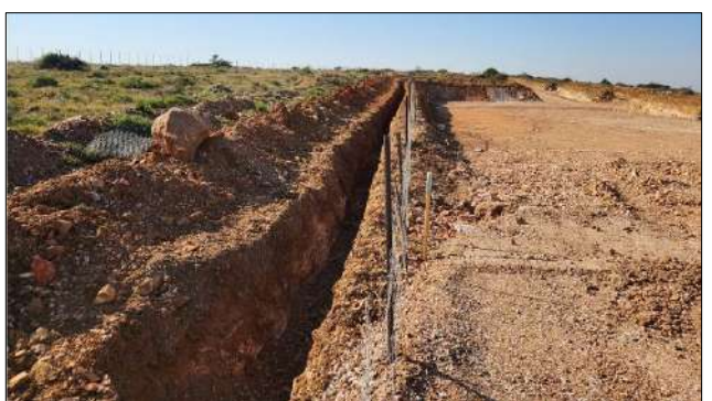
Photo 5a: MVA cables still to be installed in trench.
