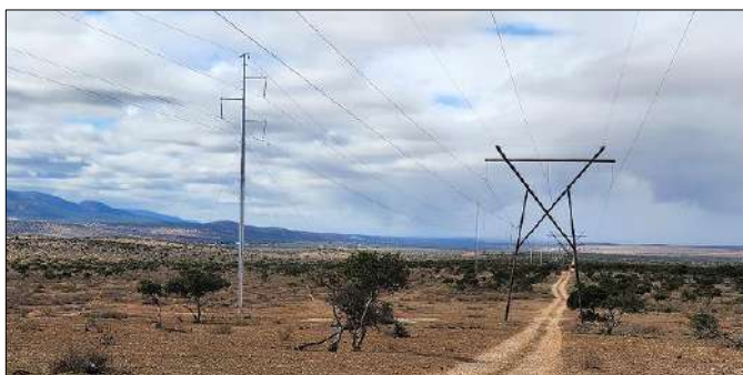
Photo 7c: View east along a strung section of the SW powerline on the Glenconnor farm portions.
