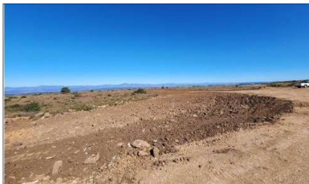
Photo 2a: State of rehabilitation, topsoil levelling underway.
