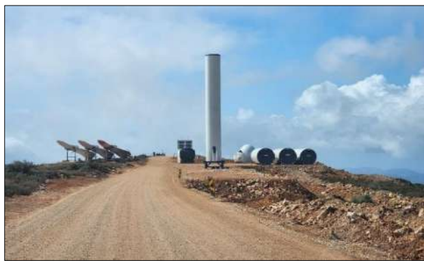
Photo 6a: Progress at wind turbine WEA10.
