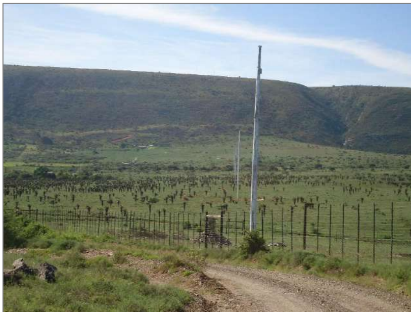
Figure 9: 13km OHPL structures.
