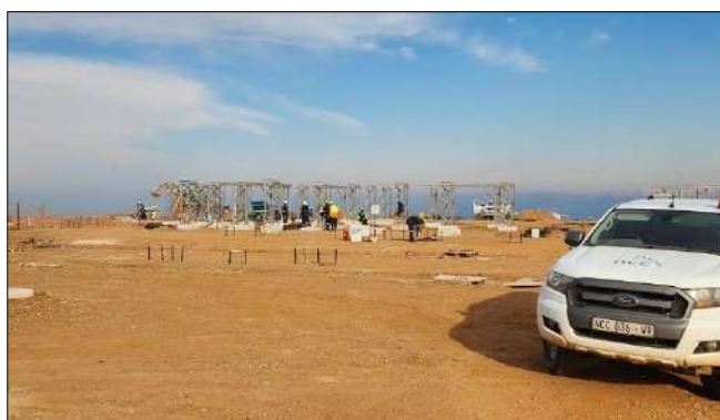
Photo 4a: Civil construction underway at the WEF substation.
