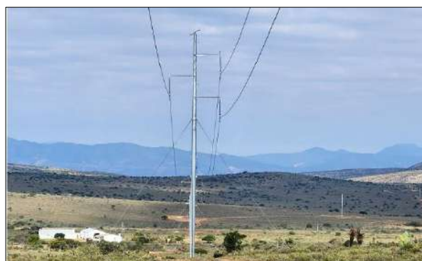
Photo 8c: View south of the strung section of powerline.
