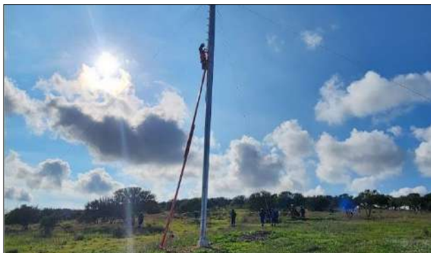
Photo 1d: Stringing preparations (dressing) at tower 143.
