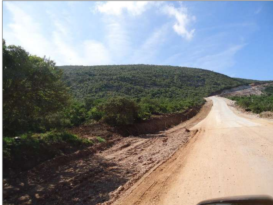
Figure 3: Arrestor bed under construction on the access road to the WEF.
