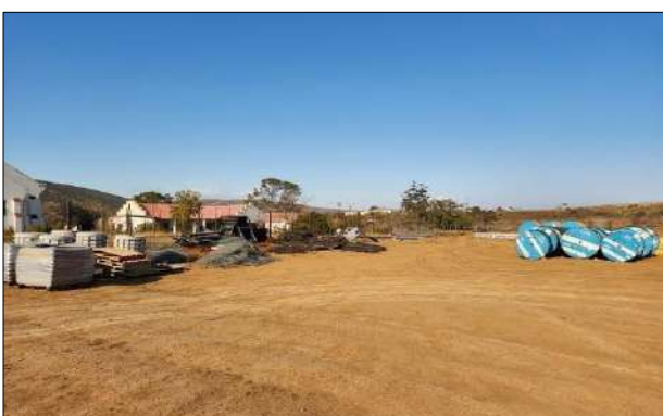
Photo 6b: Good housekeeping observed at the Wolwefontein laydown area.
