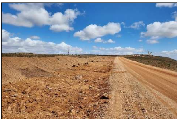
Photo 15a: Backfilled MVA trench adjacent to the road.
