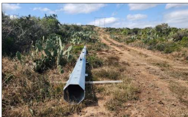
Photo 2c: Steel monopole section on site for tower CR112.
