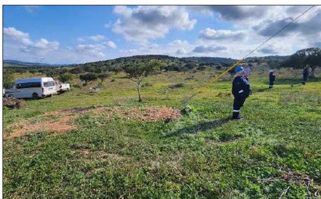
Photo 3d: Backfilled anchor stay foundation, T143.
