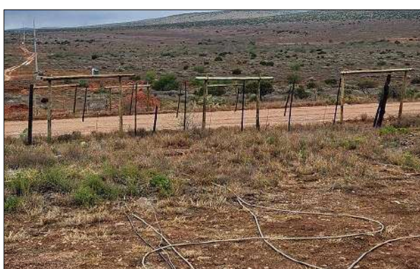
Photo 6d: Fence protective structures have been installed in preparation for stringing activities.
