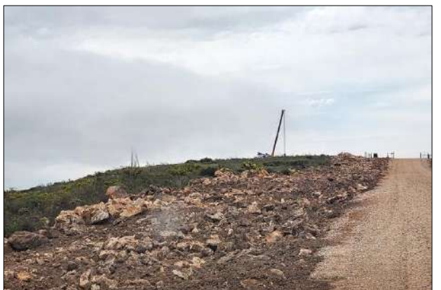
Photo 7b: Backfilled / levelled MVA cable trench adjacent to road.
