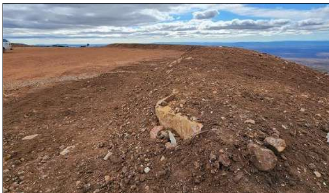
Photo 1a: Rehabilitation progress, topsoil levelled around turbine hardstands.
