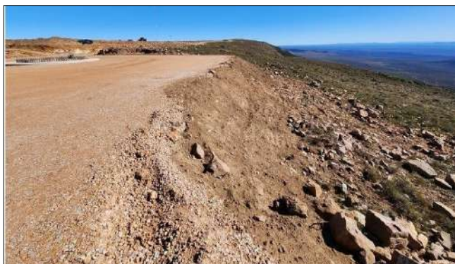
Photo 1a: Topsoil returned to sloped edges of batters.
