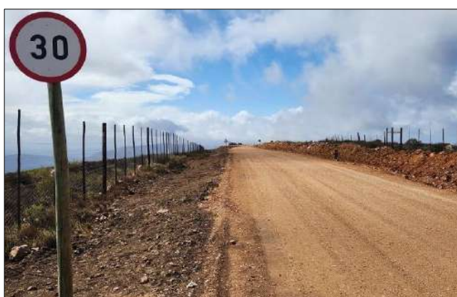
Photo 16a: Topsoil has been returned and levelled around the verges of completed road sections.
