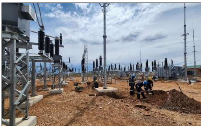
Photo 7a: Earthing underway at Lupo (switching) substation.
