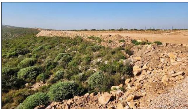
Photo 1a: Current state of ground conditions along edge of the turbine hardstands.
