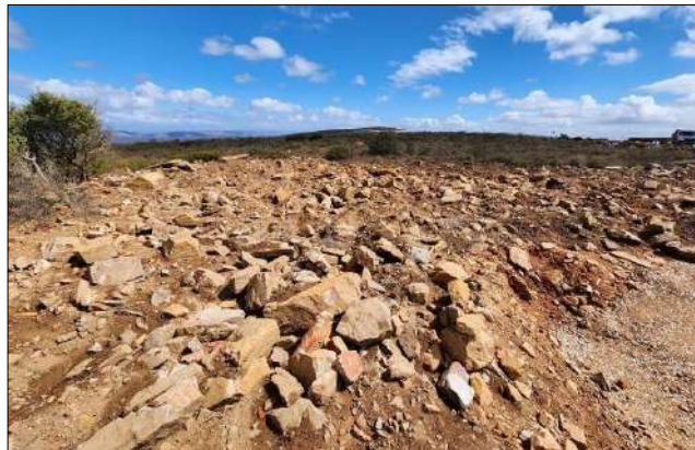
Photo 2a: Soil and rock material levelled around WEA28 hardstand.
