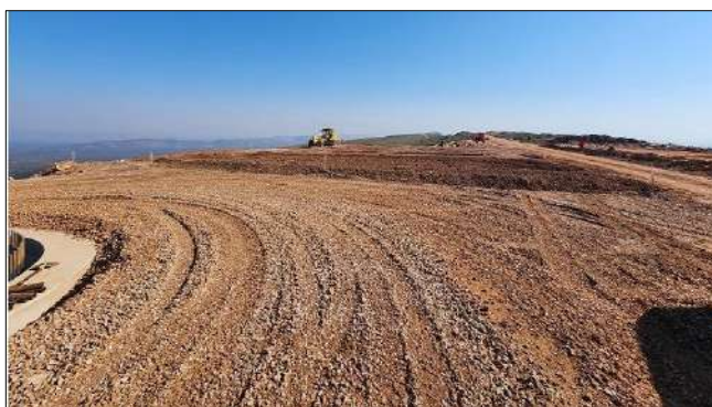
Photo 7a: Earthworks underway around one of the hardstands.
