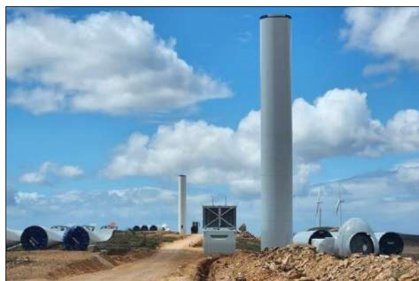
Photo 12a: Progress at wind turbine WEA08.
