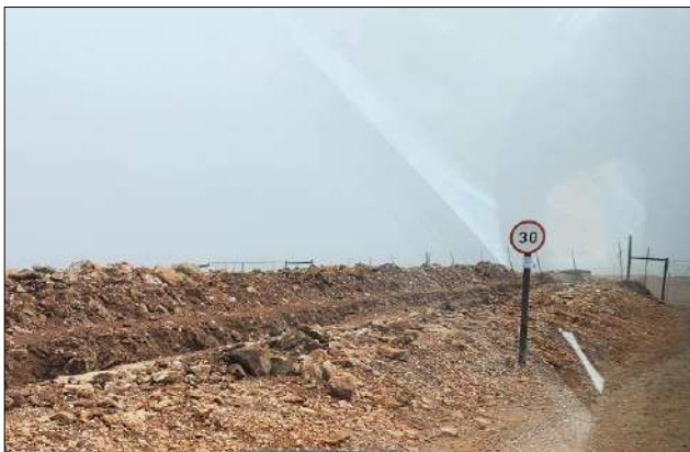
Photo 2a: Incomplete section of MVA cable trench.
