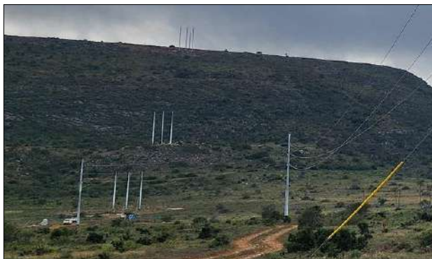
Photo 1c: & Photo 2c: Stringing of conductor cables aided with pilot cables observed to be underway.
