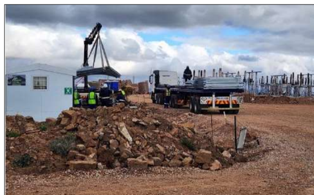
Photo 6a: Civil construction continues at the WEF substation.
