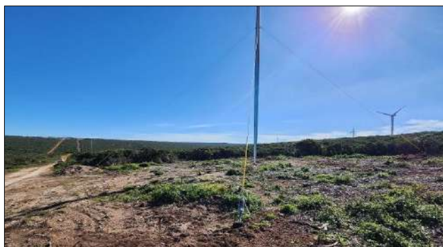
Photo 8d: Natural vegetation growth around tower CR53.
