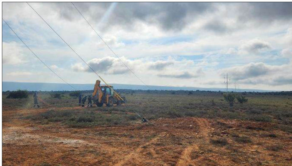
Photo 1c & Photo 2c: Preparation for stringing of conductor cables using pilot cables observed underway.
