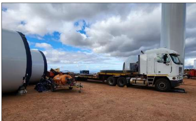
Photo 5a: Turbine components on site, drip trays in use.
