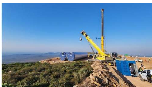
Photo 3a: Delivery of turbine components underway.
