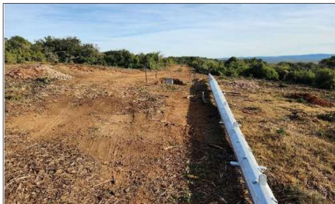
Photo 2d: Foundations still to be undertaken at tower CR178.
