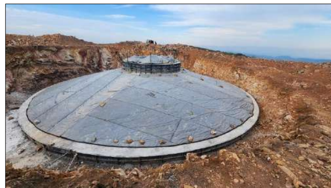
Photo 8a: Curing blanket on one of the concrete foundations.
