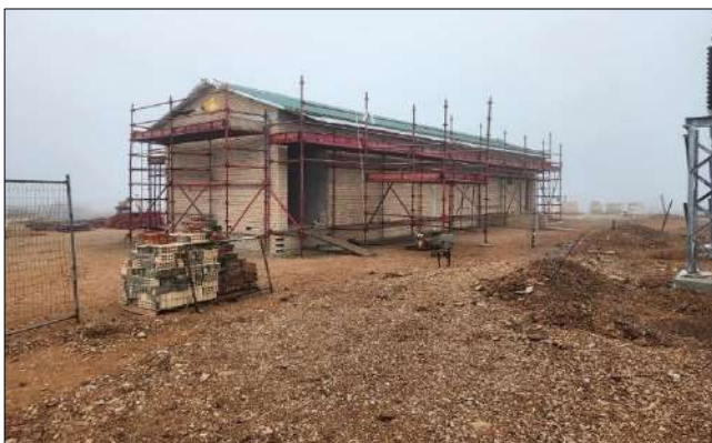
Photo 6a: Civil construction progress at substation building.
