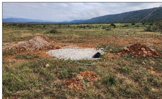
Photo 6c: Backfilling underway for the tower anchor stays.
