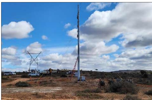
Photo 5c: Stringing activities underway along the SW line.
