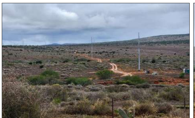
Photo 7d: Stringing activities on the Wolf-Skilpad line.
