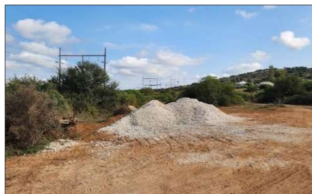
Photo 4d: Imported G5 material to replace the original yet unsuitable in-situ soil to be used as backfill material.
