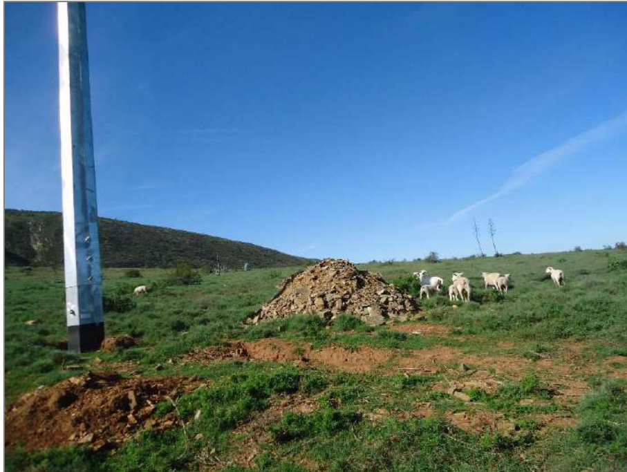
Figure 7: Stockpiles of soil along the 13km OHPL.
