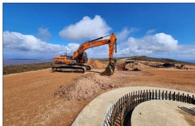
Photo 4a: Excavations underway to link MVA cables in the trench to the turbines.
