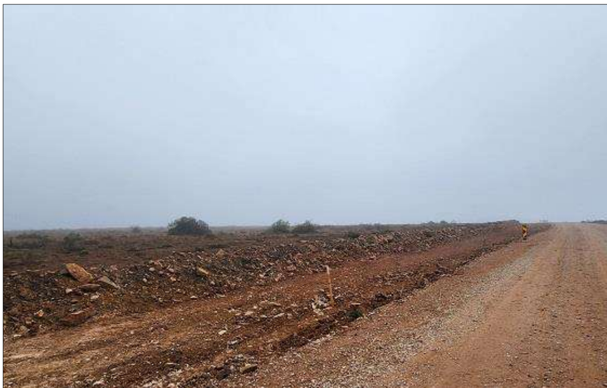
Photo 2b: Gravel section of the WEF access road where levelling of subsoil and topsoil is still to be undertaken.
