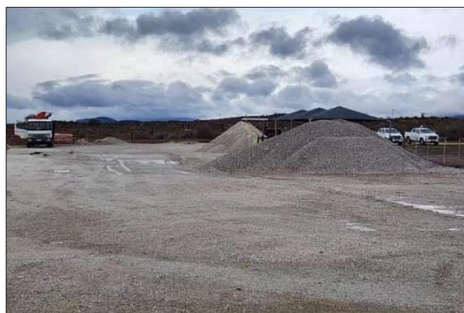
Photo 4c: Leftover G5 material from the demobilised batch facility at the Concor site offices.
