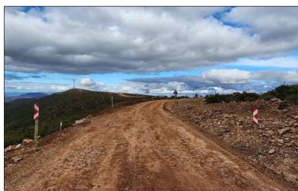
Photo 6b: Backfilled MVA trench section along road verge.
