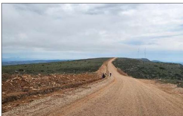
Photo 2b: Cable trench adjacent to road, to be backfilled.
