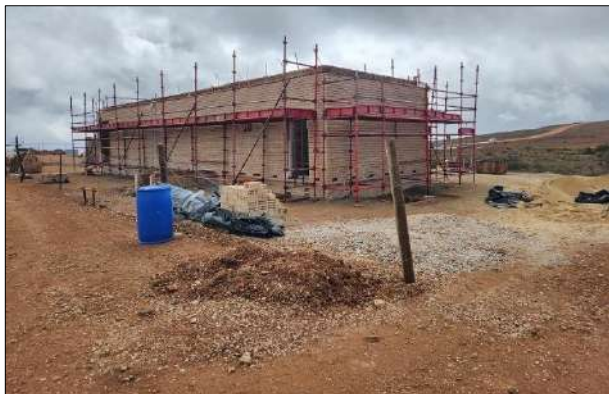
Photo 9a: Civil construction progress at WEF substation.
