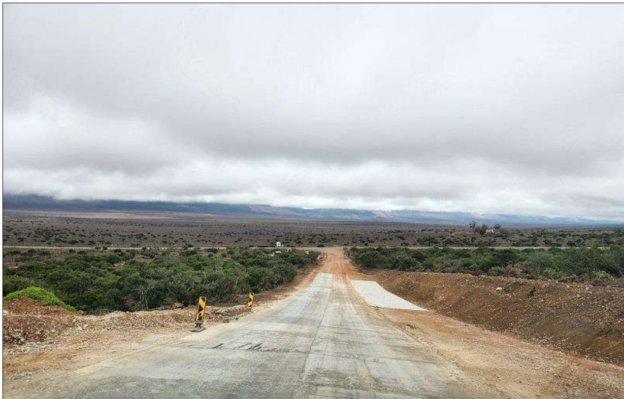
Photo 3b: Arrestor bed at the bottom of the WEF access road. Note the main tar road (R75) in the background.
