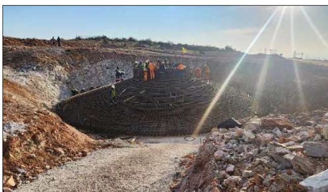
Photo 3a: Steelwork underway at a turbine foundation.
