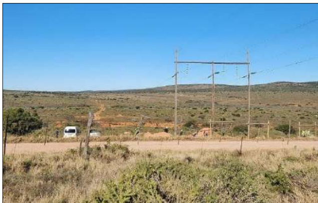
Photo 1c: WK4R excavations underway adjacent to the existing 132kV line.
