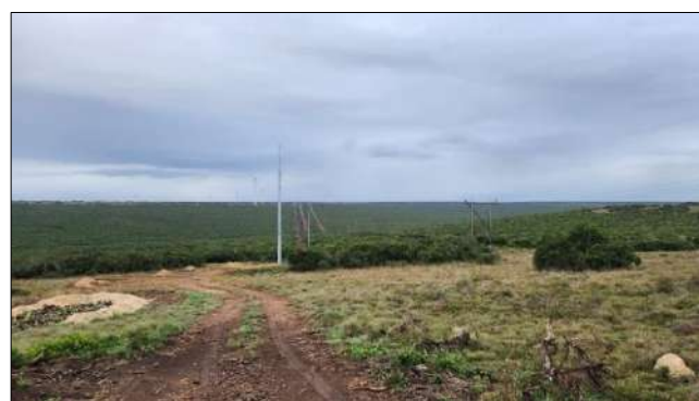
Photo 4d: View of servitude south towards Grassridge SS.
