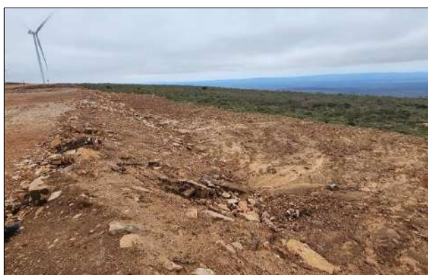
Photo 3a & Photo 4a: Small-scale soil erosion observed around several WTG hardstand edges due to recent heavy rainfall.
