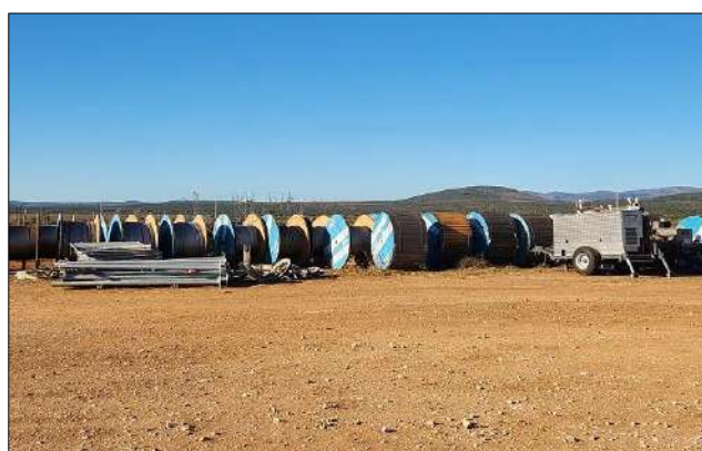
Photo 6c: Conductor drums and hydraulic stringing machine observed at the Mayogi site office.
