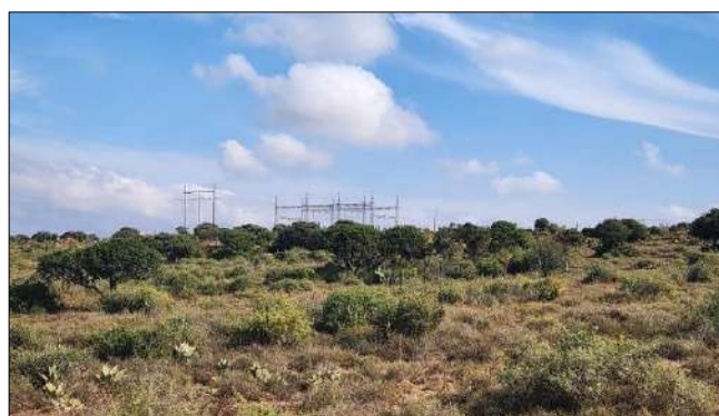
Photo 6c: Construction activities within the Wolf Substation yard have not yet commenced.
