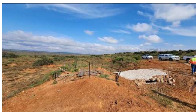
Photo 5c: Temporary crossing across an episodic drainage line to a tower position.
