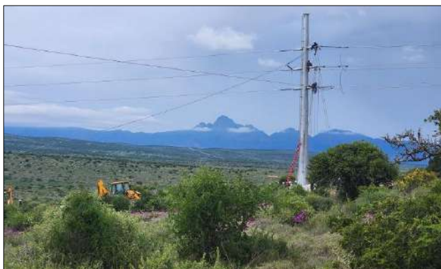
Photo 1d: Regulating underway at WK4 outside Wolf SS.
