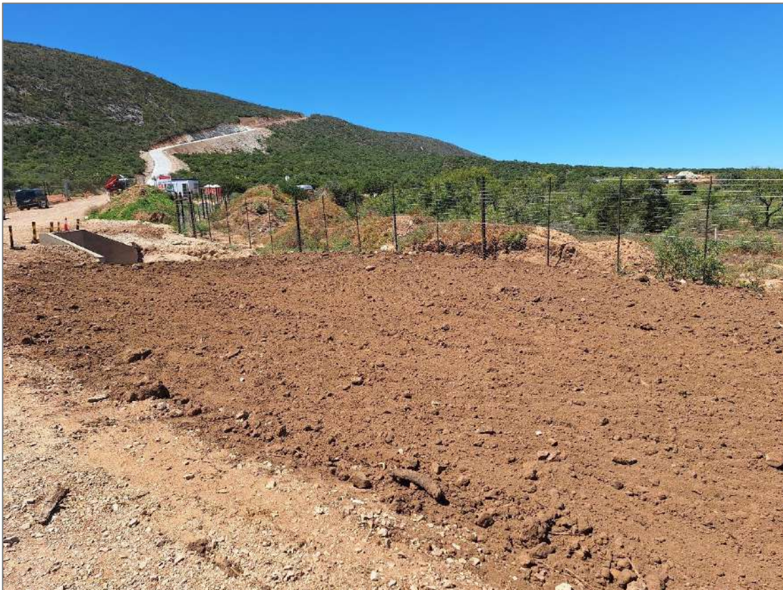
Figure 8: Topsoil being placed on slopes for rehabilitation.
