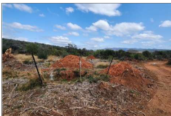
Photo 3c: Barricaded excavations at CR144A.
