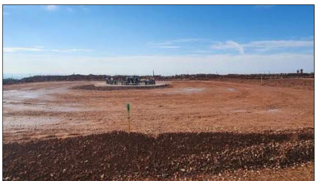
Photo 5a: Backfilled foundation and turbine hardstand.
