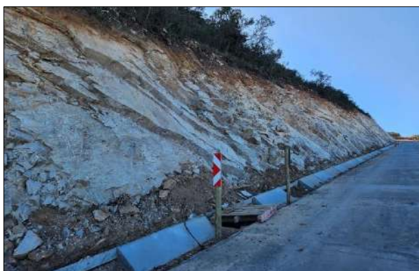
Photo 6b: Stormwater v-drains between road and cut slope.
