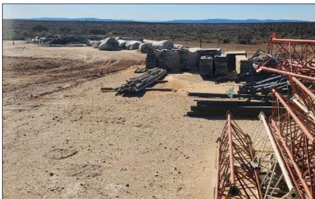
Photo 2b: Neat, tidy housekeeping observed on site.
