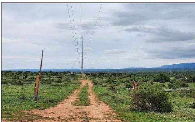
Photo 2d: Remnants of the dismantled/broken down timber pylons along the former Skilpad-Wolf 132kV powerline.
