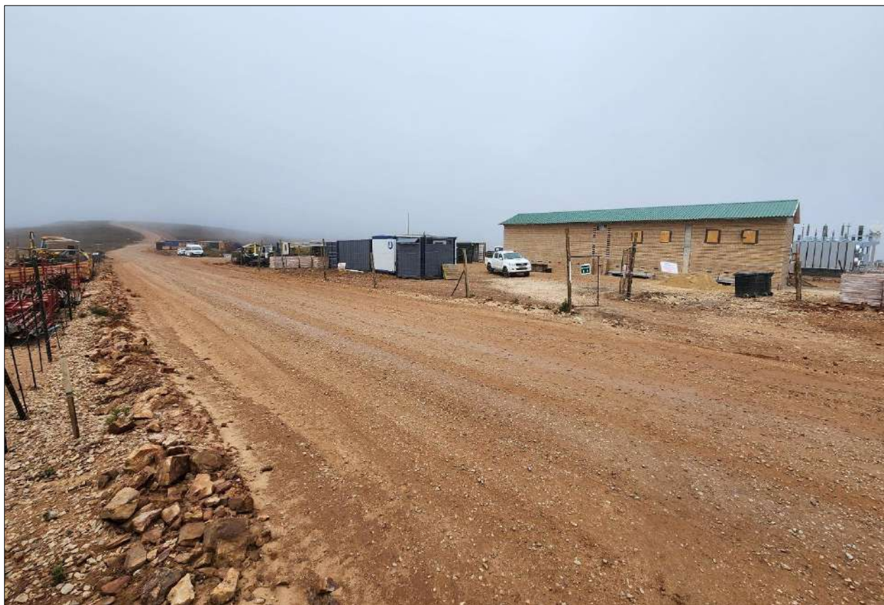
Photo 1b: Gravel section of the WEF access road passing the substation.
