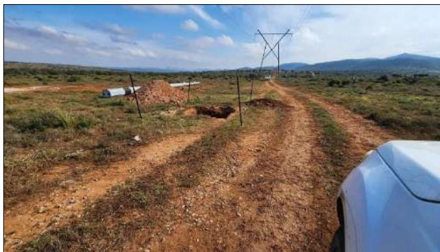
Photo 1d: Barricading in place for open excavations.
