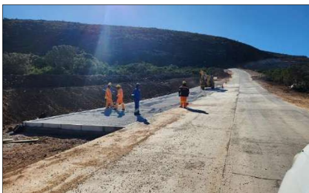
Photo 5b: Construction of arrestor bed for the road underway.
