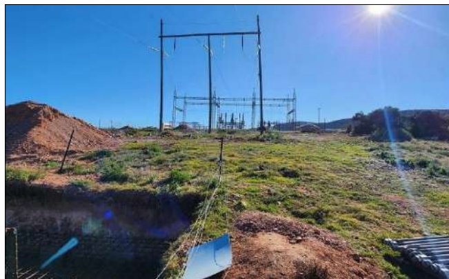
Photo 2c: WK3 tower excavations underway outside Wolf SS.
