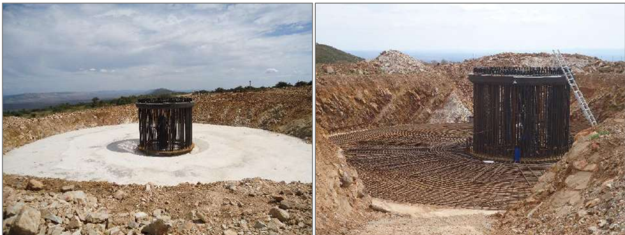
Figure 6: Concrete pouring work in progress.
