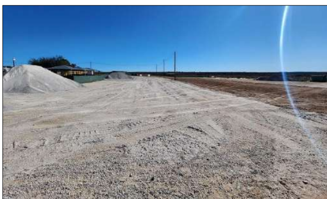
Photo 3b: Concrete batch plant has been demobilised.
