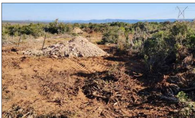
Photo 3c: Barricaded excavations at CR202.
