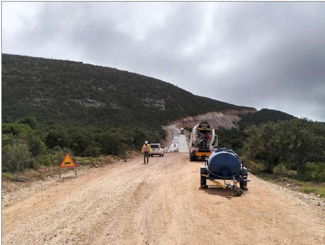
Figure 6: Concrete on the Main access road.
