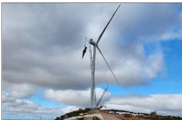
Photo 7a: Wind turbine (WEA09) being assembled.
