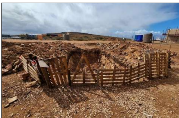
Photo 11a: Construction of transformer oil dam underway.
