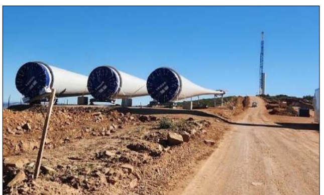
Photo 3a: Delivery of turbine components continues.
