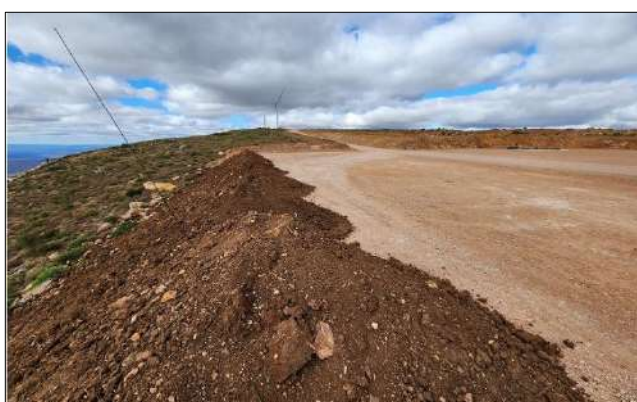
Photo 3a: Topsoil returned to sloped edges of batters.
