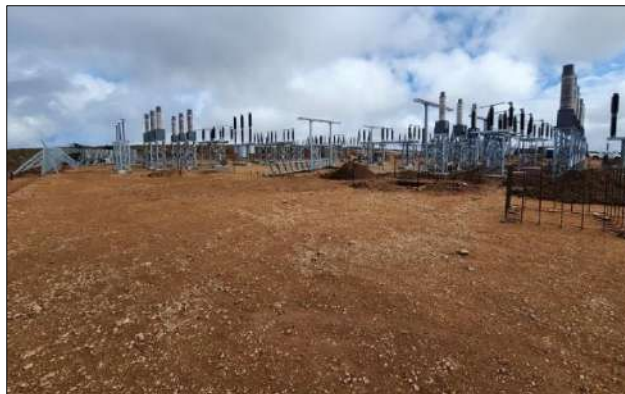
Photo 10a: Civil construction progress at WEF substation.
