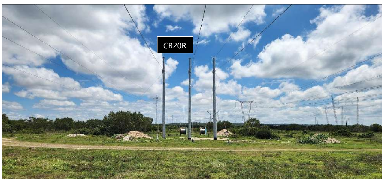
Photo 3d: Stringing completed on the Grassridge-Skilpad powerline between tower CR20R and Grassridge Substation.
