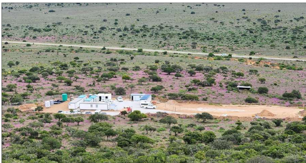
Photo 5c: Vestas office block adjacent to Concor's previous laydown / refuelling area.
