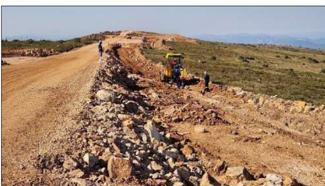
Photo 6a: Backfilling a section of MVA cable trench underway.
