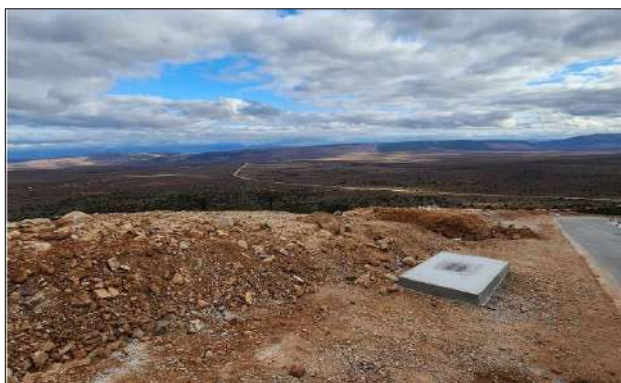
Photo 7b: Drainage installation along the road's fill slope.
