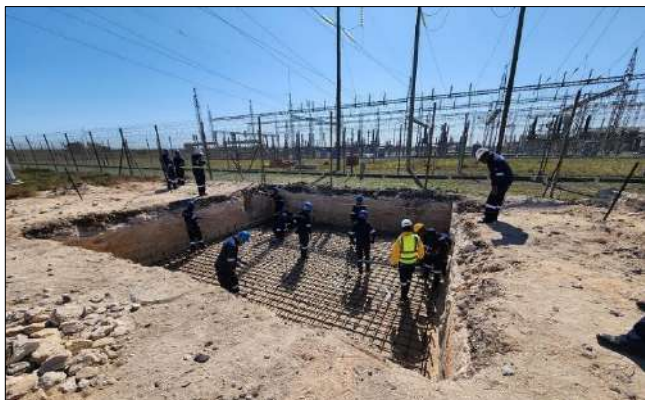
Photo 1c: Rebar installation in preparation for concrete foundations at CR2 outside Grassridge SS.
