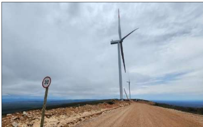
Photo 1a: Assembled wind turbine generators ("WTGs").
