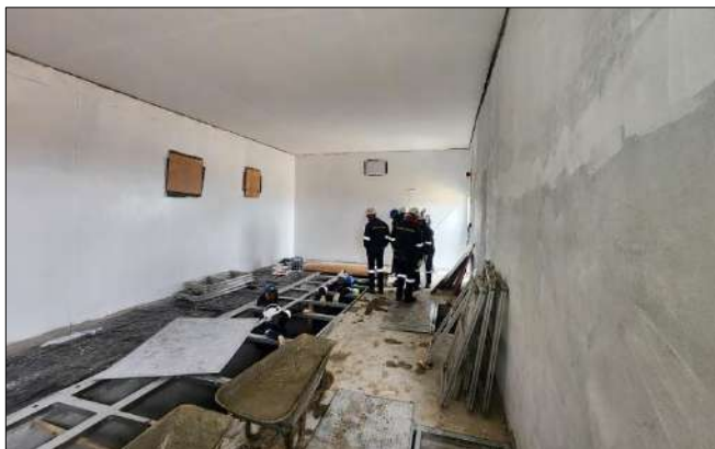
Photo 7a: Painting underway in (switching) substation building.
