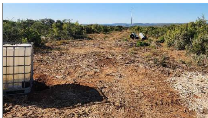
Photo 4c: Steel tower components delivered to servitude prior to erection of CR202.
