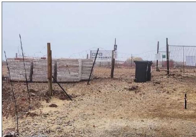
Photo 10a: Bricks stored at the substation laydown area.
