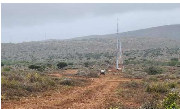
Photo 8d: Stringing done up to and backstayed at tower WK5.
