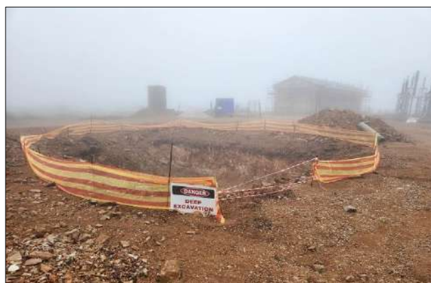
Photo 4a: Construction of transformer oil dam underway.
