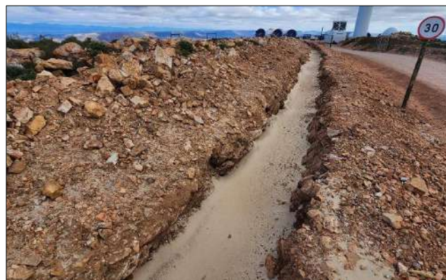
Photo 4a: Section of MVA cable trench still to backfilled.
