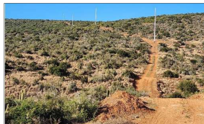
Photo 4d: Access route with berms between CR157 & CR154.
