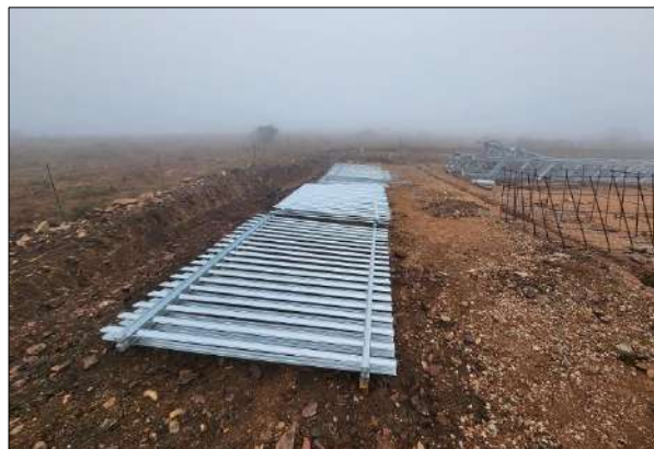
Photo 8a: Construction of steel fencing around substation.
