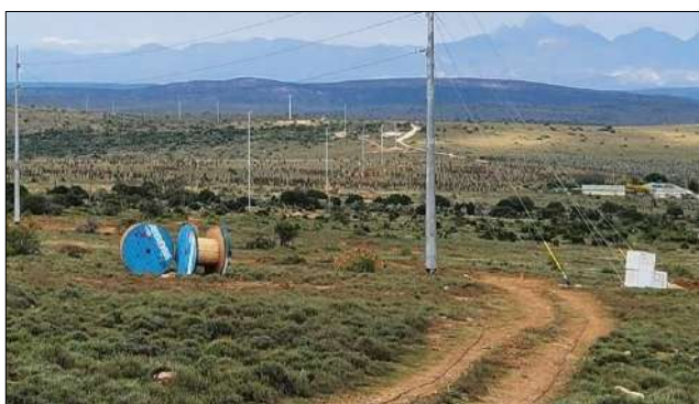
Photo 3c: Back-stayed tower. Stringing to be completed once construction of the WEF substation advances further.
