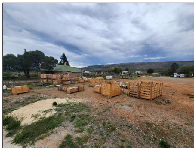
Photo 4c: Good housekeeping observed in the Wolwefontein material storage / laydown area.
