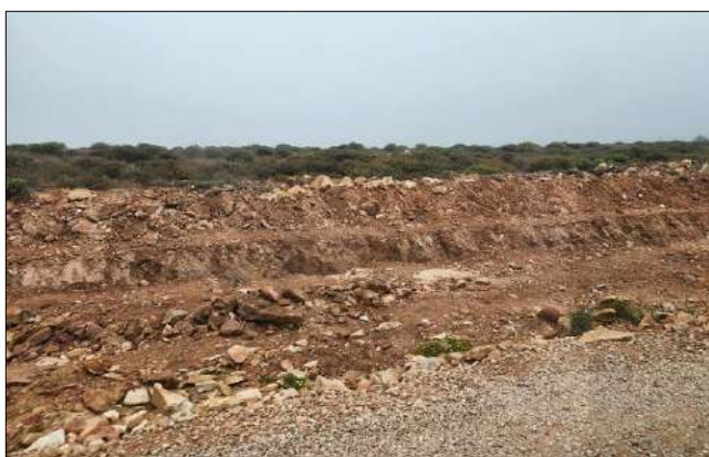
Photo 3a: Excavated MVA cable trench requiring completion.
