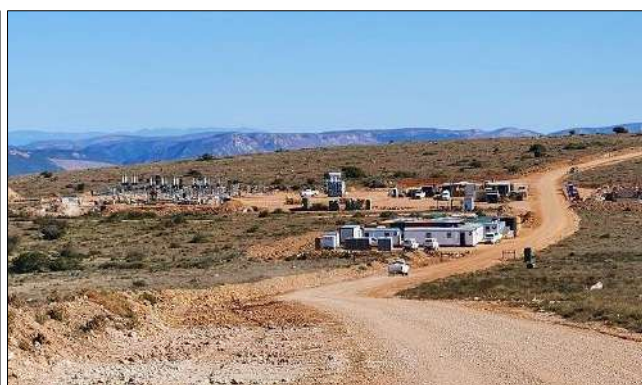
Photo 6a: Civil construction continues at the WEF substation.
