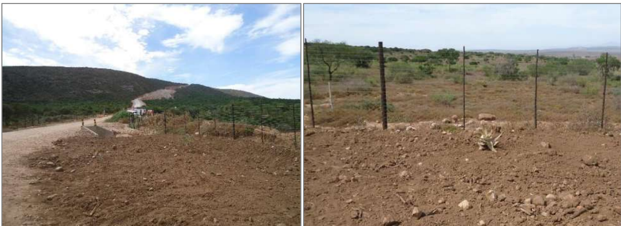
Figure 7: Rehabilitation at bellmouth.
