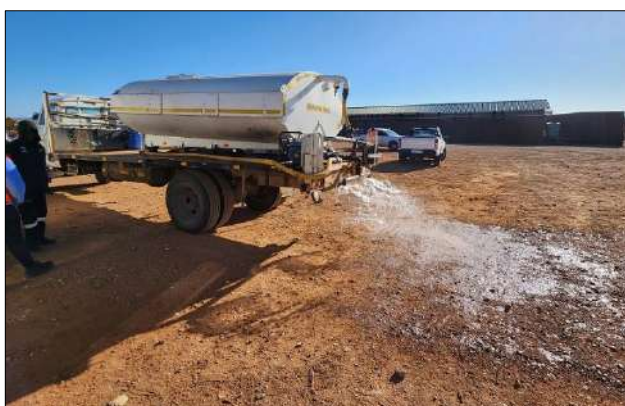
Photo 3b: Dust suppression observed at site camp.
