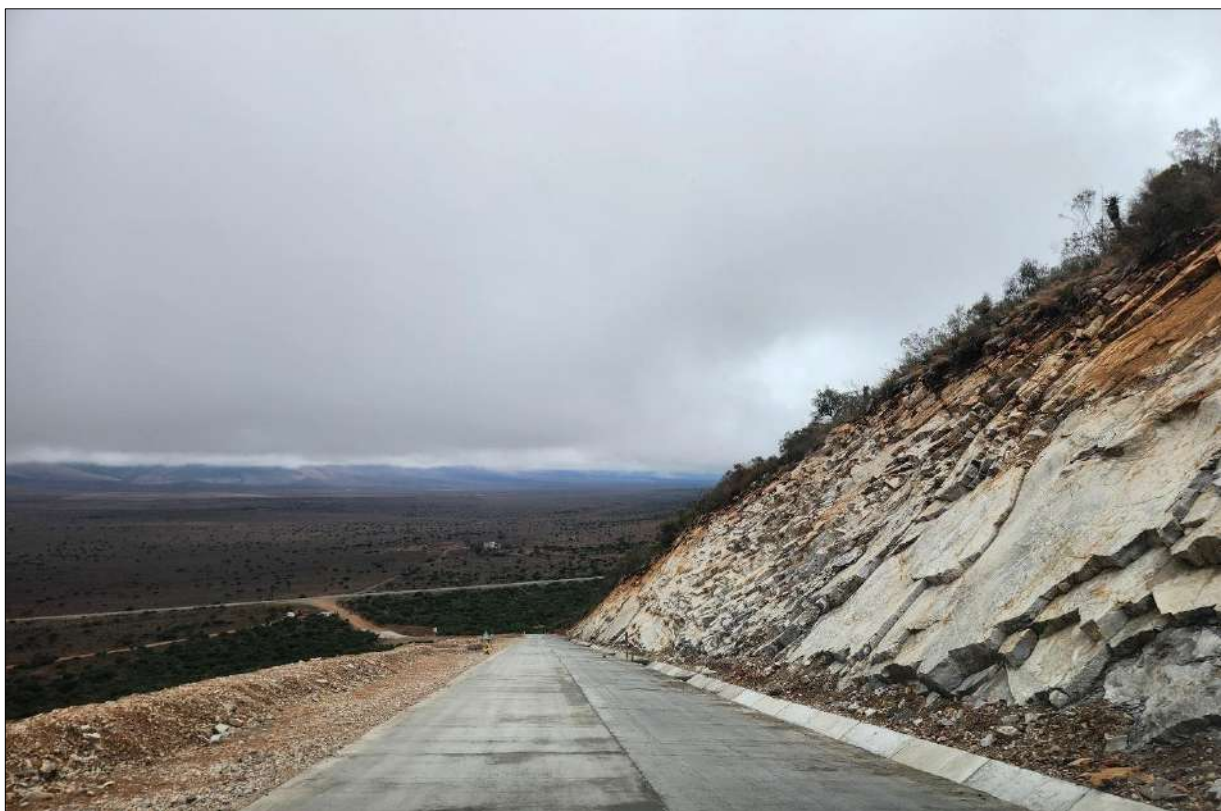
Photo 4b: Tared section of the WEF access road accessible via the R75 main road between Kleinpoort and Jansenville.
