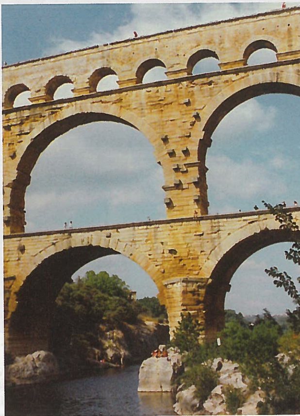
The aqueduct that crosses the Gardon River was once attributed to the Pantheon's architect. Protruding stones on the face supported scaffolding.
