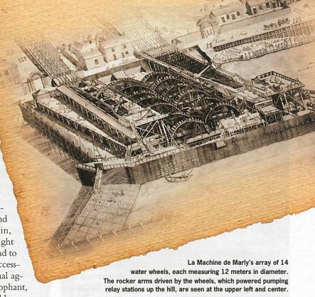
pumps, the water wheels, by means of a bizarre assortment of levers and bell cranks, provided an oscillating pull to pairs of chains that relayed power up the hill.
