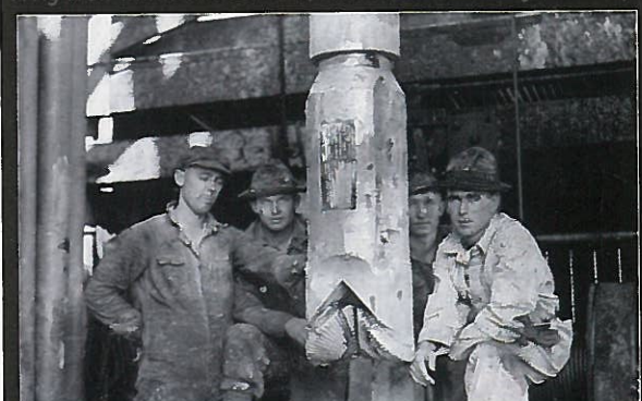
A rig crew with a two-cone bit, a landmark in drilling efficiency.
