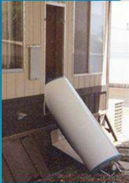
During an earthquake, an unbraced water heater can topple, which can start a fire or lead to major water damage.
