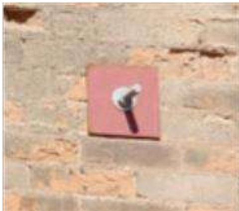
A steel plate with anchor bolts.
