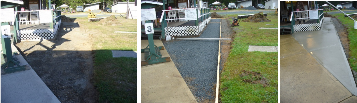
Concrete sidewalk next to the Club House – earthworks, formwork & poured concrete
