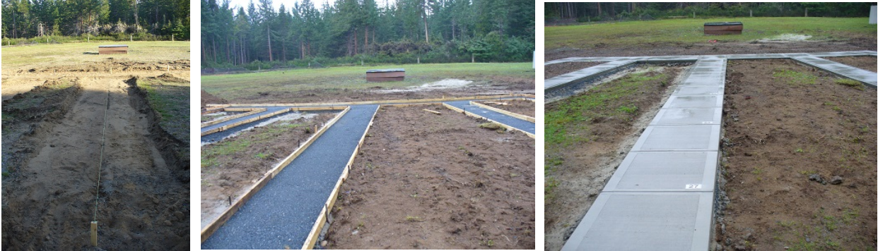
Shooting Station #2 Close-up – earthworks, formwork & poured concrete
