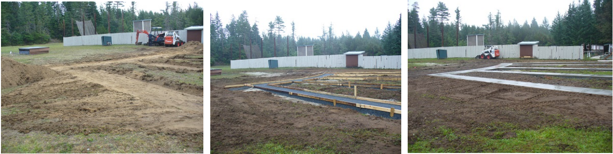
Shooting Station #2 – earthworks, formwork & poured concrete
