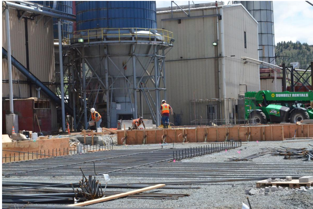
Construction workers complete concrete forms and metal reinforcement for one of the foundations for the torrefaction plant at the Malheur Lumber Co. plant in John Day.
