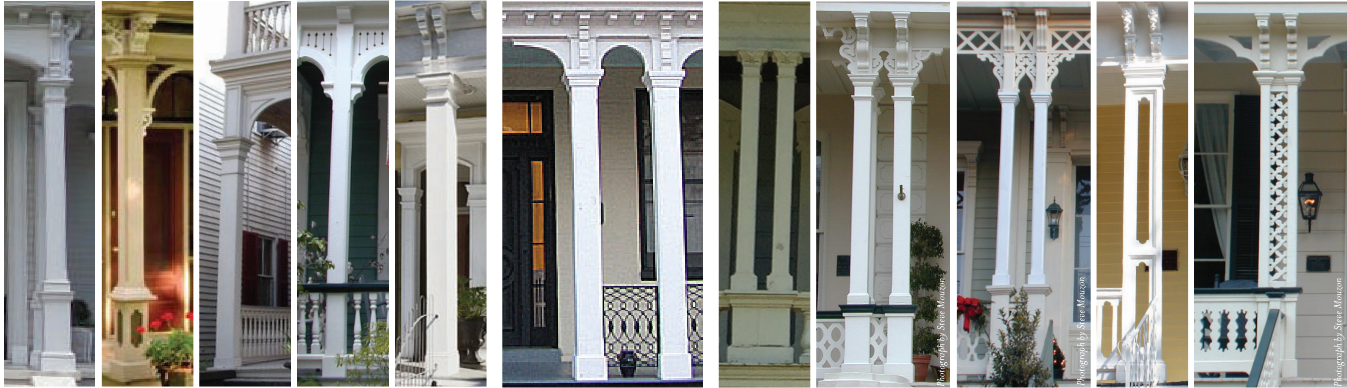
Columns are square, often on a handrail-height base. Columns are also often chamfered, but never round (like Victorian). Brackets, single or paired, often sit atop columns. Beams are segmented arches, or, when flat, often have arched scrollwork/trimwork.
