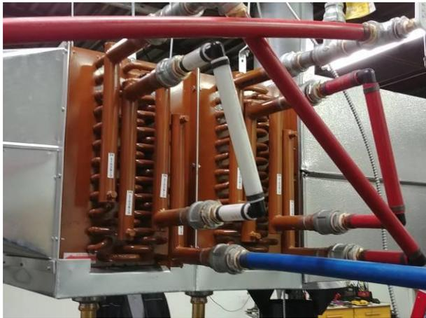
*FGR heat exchanger and connections*
