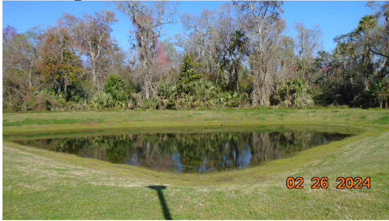
Pond 4: Pond was in good condition. The water level is low.
