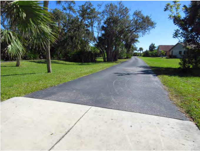
GENERAL VIEW OF ASPHALT ACCESS DRIVE
