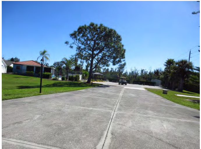
GENERAL VIEW OF CONCRETE PAVEMENT
