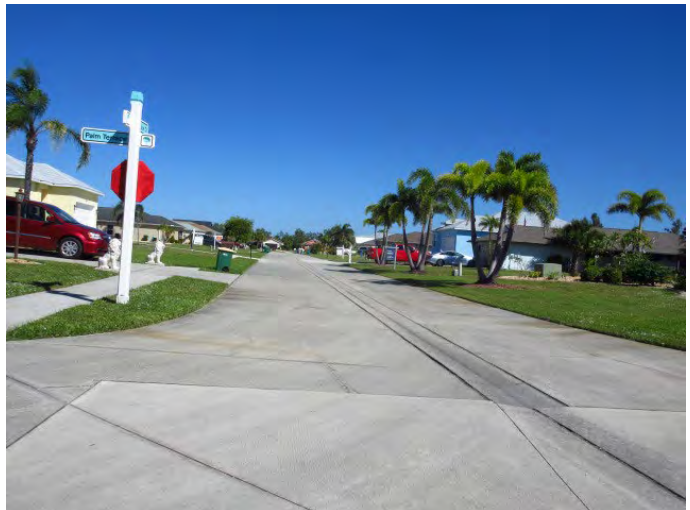
VIEW OF CONCRETE PAVEMENT
