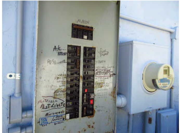
VIEW OF ELECTRICAL EQUIPMENT
