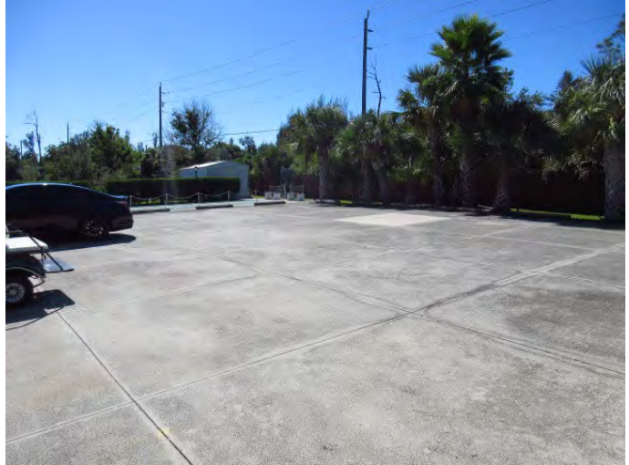
GENERAL VIEW OF PARKING AND PAVEMENT
