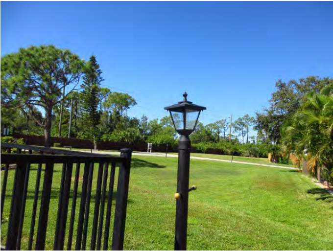
GENERAL VIEW OF SITE LIGHTING
