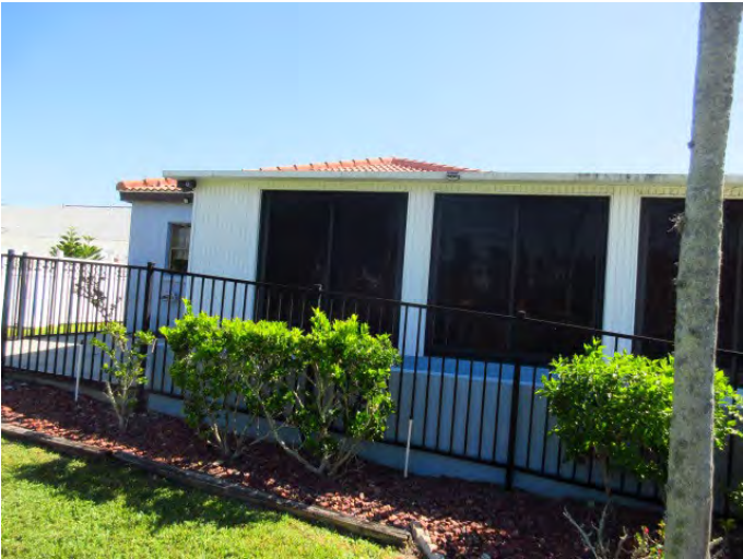
VIEW OF BUILDING EXTERIOR FINISHES
