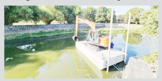
The Department of Environment and Natural Resources (DENR) recently turned over four backhoes-on-barge to the Department of Public Works and Highways (DPWH) to aid in the desilting, dredging, and hauling of solid waste from the Muntinlupa-Parañaque-Las Piñas river system and its tributaries
