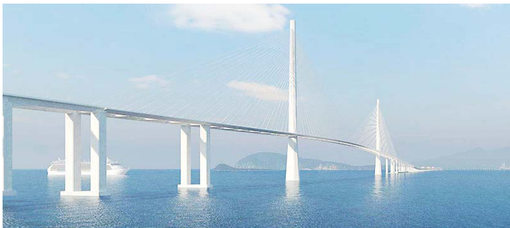
The Bataan-Cavite Interlink Bridge speeds up travel—from five hours down to just 40 minutes—between Bataan and Cavite.
