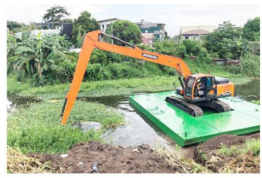
Citing the importance of dredging operations, NIA Regional Manager Lopez said the new equipment will help address the problems with siltation and improve flood control in the city due to an increase in the dam's water storage capacity.
