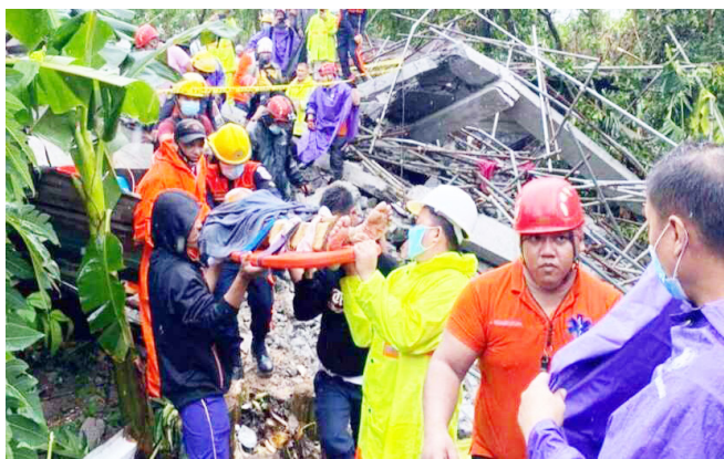
The rescue and retrieval operation at the building extension of the factory of Polytechnique Mfg., Inc. in Purok 4, Langkaan 1, Dasmariñas, Cavite Thursday night. From the Office of Representative Elpidio Barzaga of Lone District of Dasmariñas City
