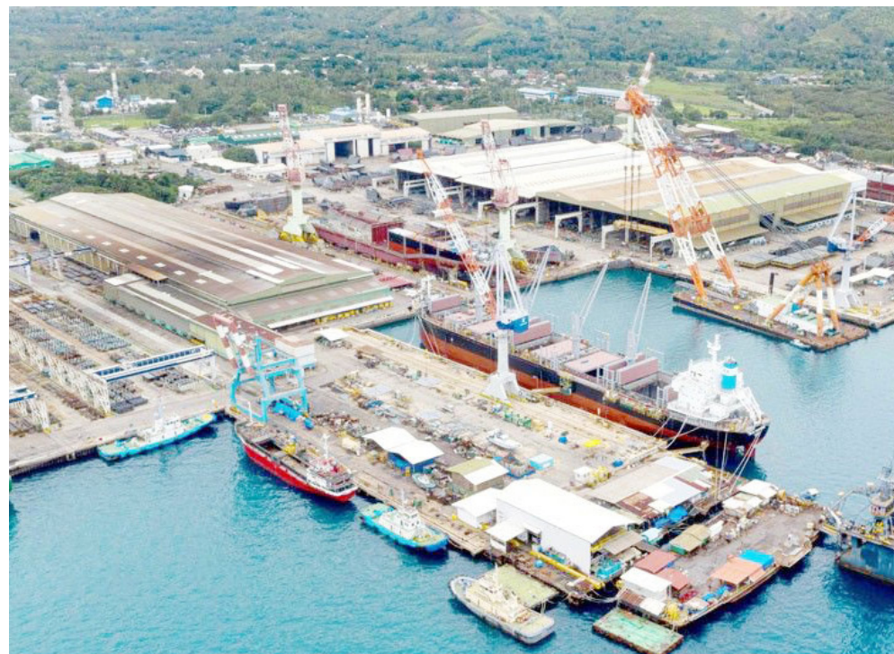
Tsuneishi Heavy Industries started developing land and construction of shipbuilding facilities in 1994. Today, it has grown to become one of the largest shipbuilding factories in the Philippines with the capacity to build about 20 vessels per year.
