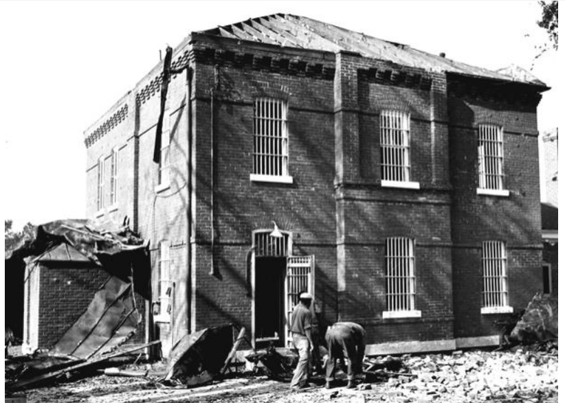
(Above) The outer brick façade was stripped off during demolition in this October 17, 1959 Daily Press photograph.
