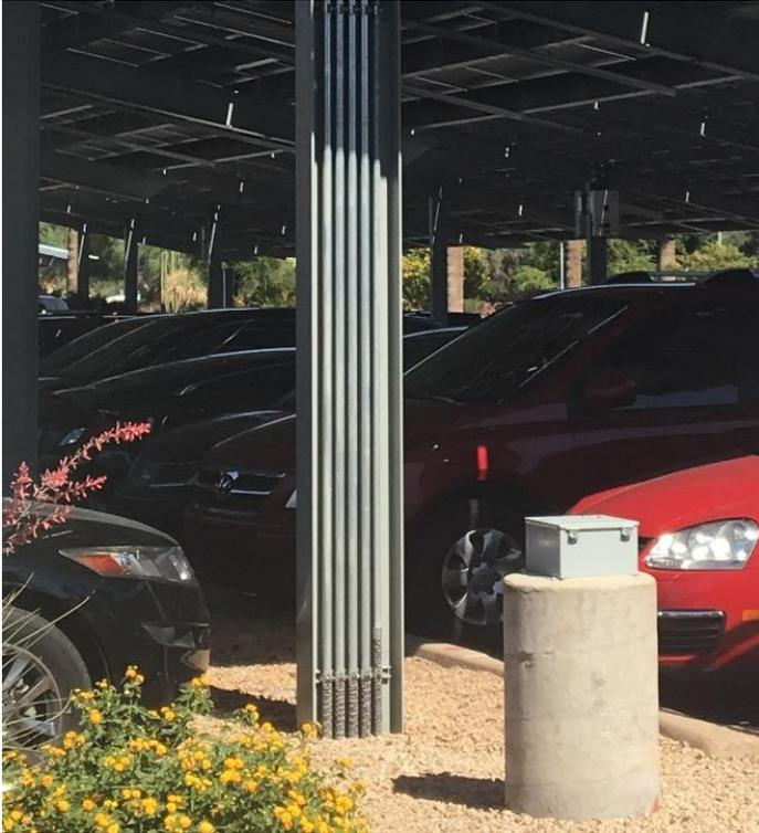
*Conduit in I-beam, and j-box directly exposed to afternoon sun.*
