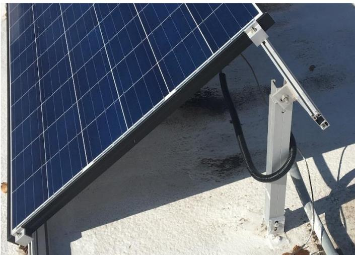
*DC wiring on edge of array protected from sun prior to entering conduit*
