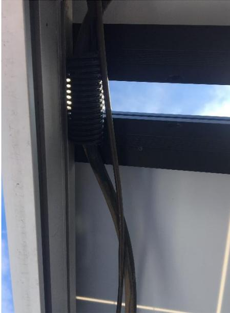
*DC wiring between modules (solar panels) protected by loom (underneath modules)*
