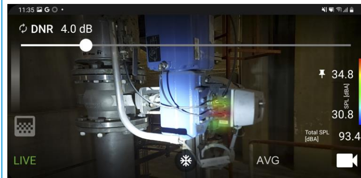
SPL AT 1M 32.8DB DISTANCE 0.8M SPL AT MEASUREMENT DISTANCE 34.8DB
