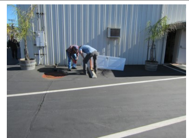
Trimming model room door
