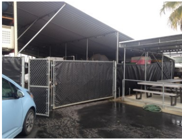
Fence cover on lean-to hangar
