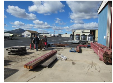
Cleaning up the south ramp
