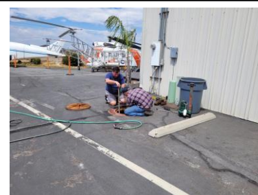
Installing new sewer pump
