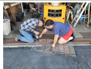
Cutting a sewer plate cover
