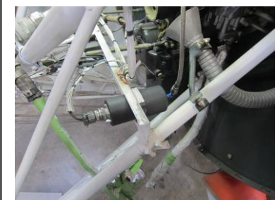
Manifold pressure transmitter
