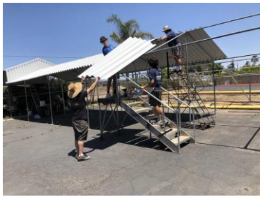
Scouts working on roof
