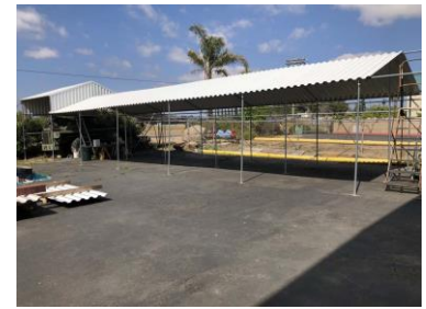
Garage/shed roof in May
