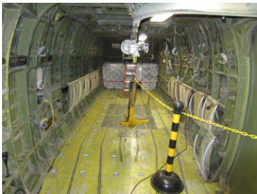
H-37 cabin deck
