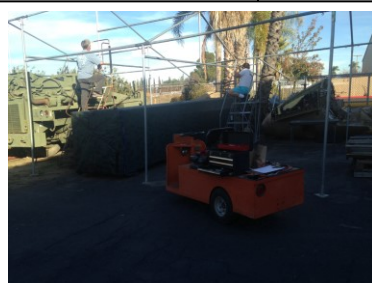
Outside storage framework
