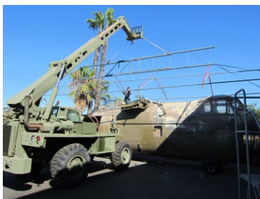
Lifting the H-37 awning cover
