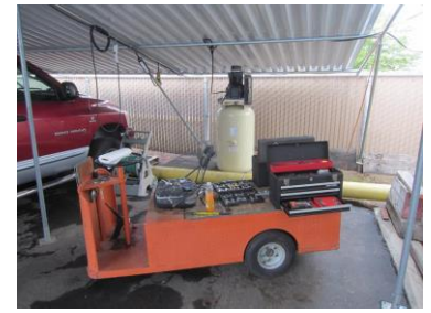
New compressor set up
