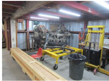
New lights installed
