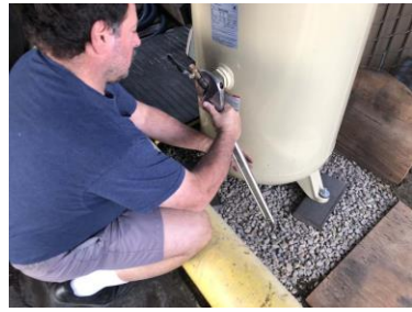
Compressor valve adjusted
