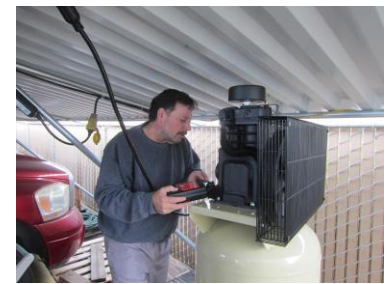
Compressor motor oil added
