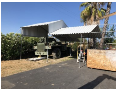
Garage roof extended
