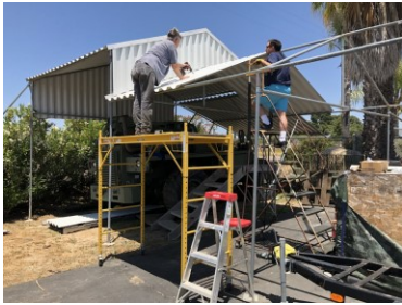
Garage roof in work
