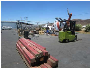
Cleaning the north ramp
