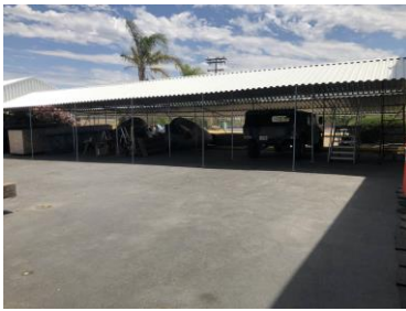
Outside parking structure
