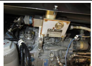
Repaired ECA installed
