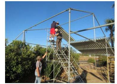
Adding on a garage roof
