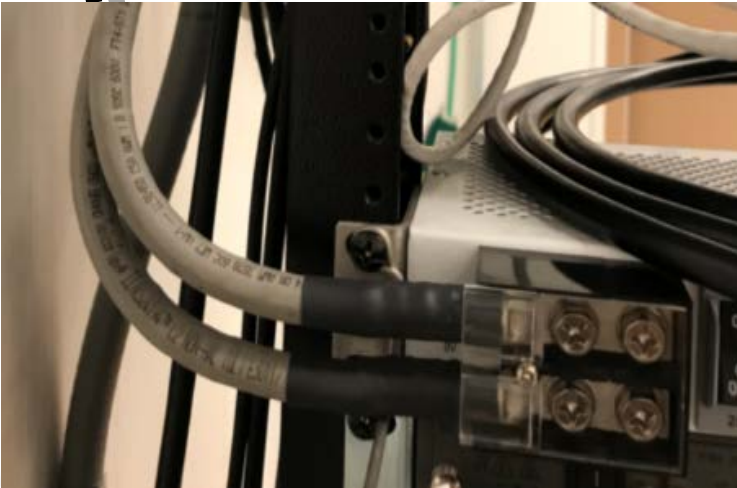
DCDU in Existing site rack
