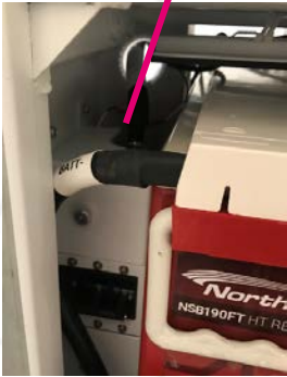
Battery Breaker/Fuse ALM
