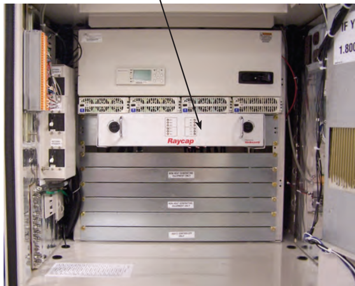
14.12 An SPD assembly mounted in a DC power and battery enclosure
