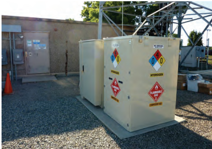
10.9 An actual fuel cell and hydrogen storage cabinet installation
