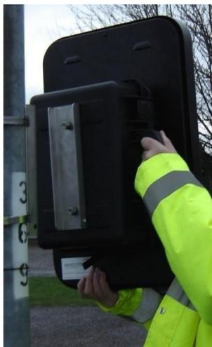
Carefully lift the sign on the bracket. The sign has two nuts that fit into the keyholes on the bracket. Once inside the keyhole, slide the sign down into the smaller part of the hole. When this is completed, the sign will be securely in place.
