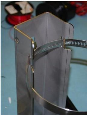
Slide the tamtorque through the two gaps in the bracket and then around the post to which the sign is being fixed onto
