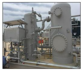
SulfurSWEET® a division of Nexo Solutions provides systems, technologies and chemicals for H<sub>2</sub>S and mercaptans removal from gas streams. The company also provides a variety of consulting, engineering and technical services along with onsite support.
