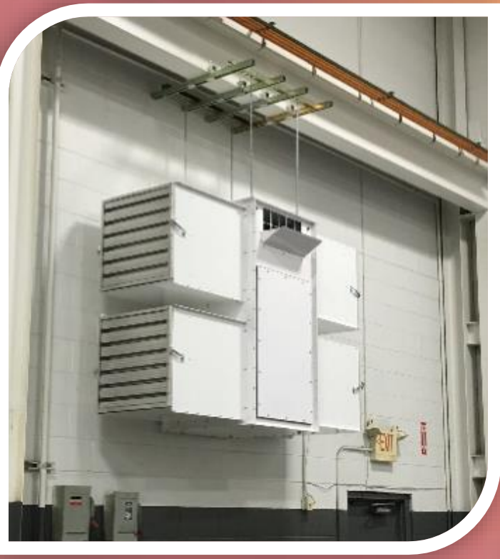
2423: Features forward facing exhaust
