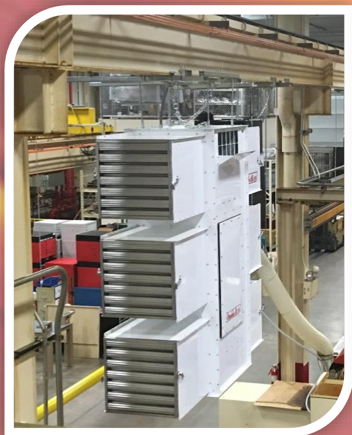
3623: features forward exhaust for ducting away from the unit
