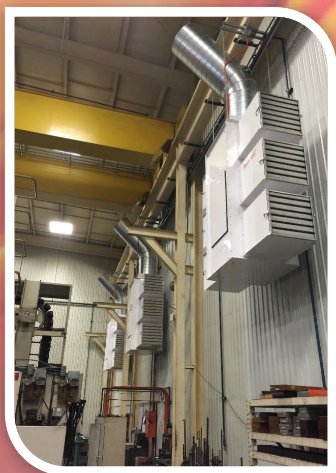
3623VT: features vertical exhaust for ducting away from the unit
