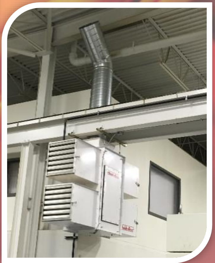
2423VT: Features vertical exhaust
