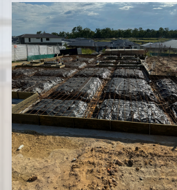
Conventional Raft Slab
