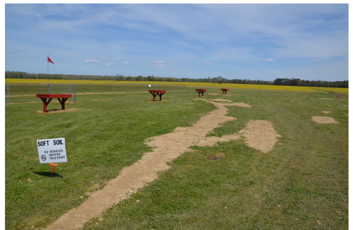
Repaired areas of the field.
