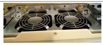
(3) Turn the fan casing in the direction of the arrow and pull it towards you.
