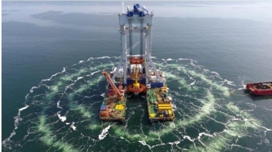
Twin curtains of bubbles surround this pile-driver during turbine foundation installation (Vineyard Wind)
