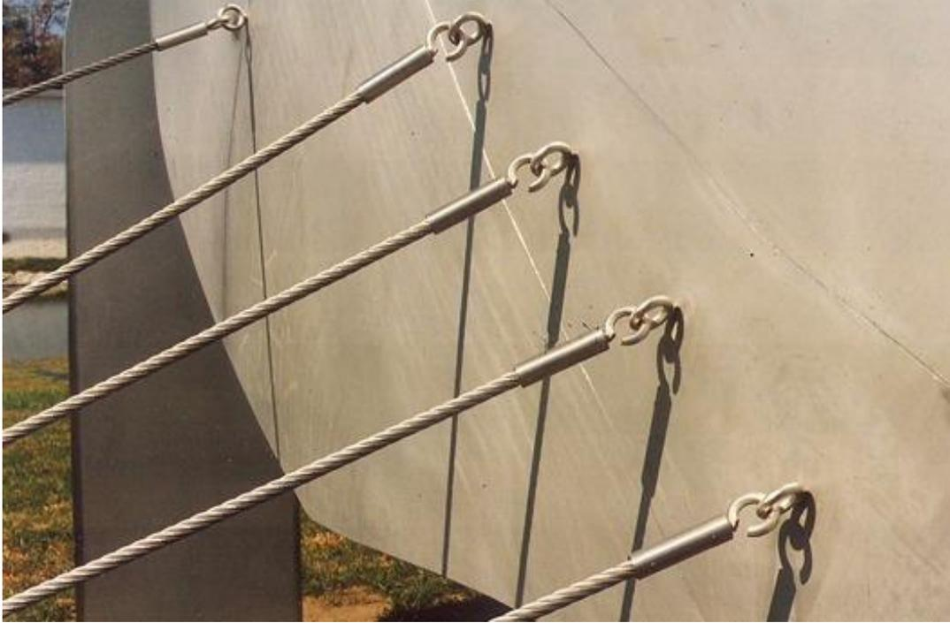
*Stainless steel wire rope and custom designed hooks with internal threads for tightening*
