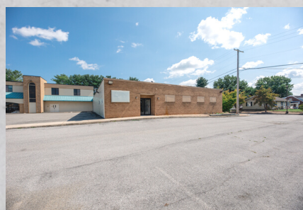
13331 PENNSYLVANIA AVE FLEX SPACE
