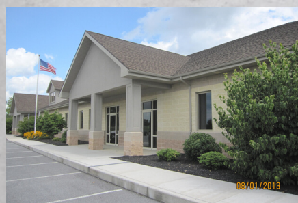
HUNTERS GREEN PARKWAY -OFFICE/WAREHOUSE
