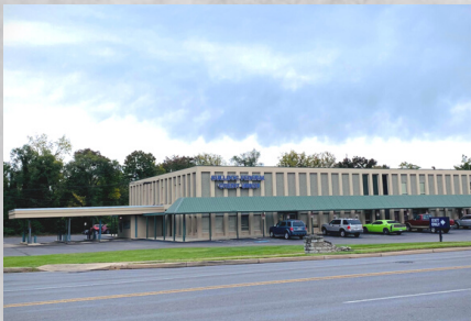
580 NORTHERN AVE -PROFESSIONAL OFFICE
