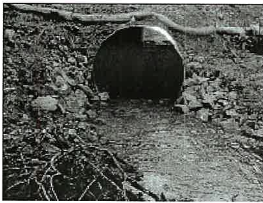
Lower Took Fish Passage Culvert. (July 2004, photo provided by the BNF)
