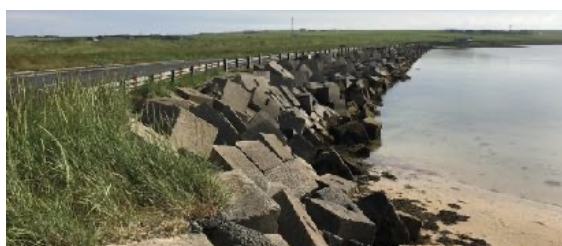
WW2 barrier No. 4 linking Burray with South Ronaldsay.
