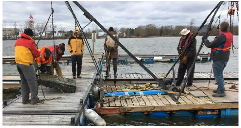
With the mud washed off, the anchor is placed on dock in order to visually inspect the condition of the shackles and chain used to secure it to the dock.
