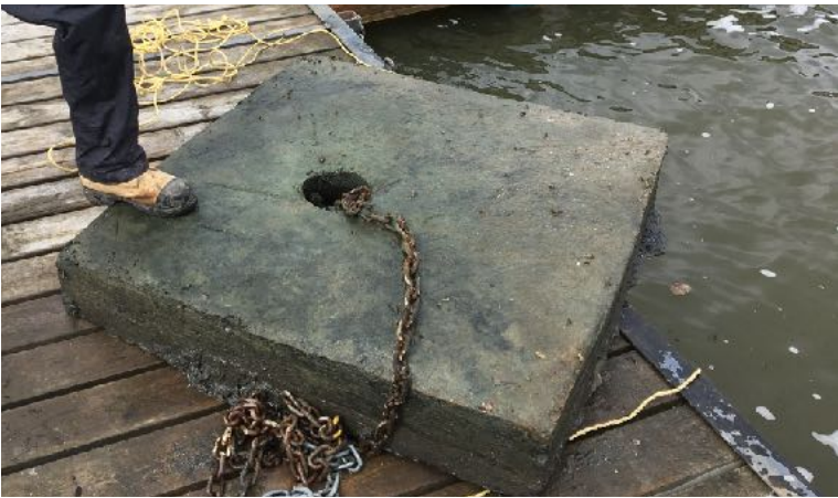
Close up of anchor shows its size in relation to Patrick's foot. This one looks fairly new and appears to be in good shape.
