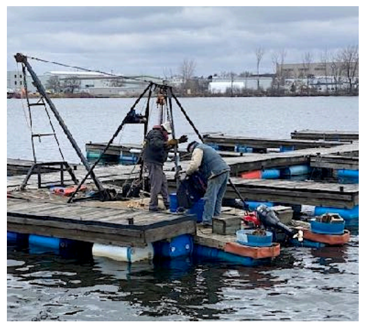
Using the crane winch at a dock to reposition one of its anchors.
