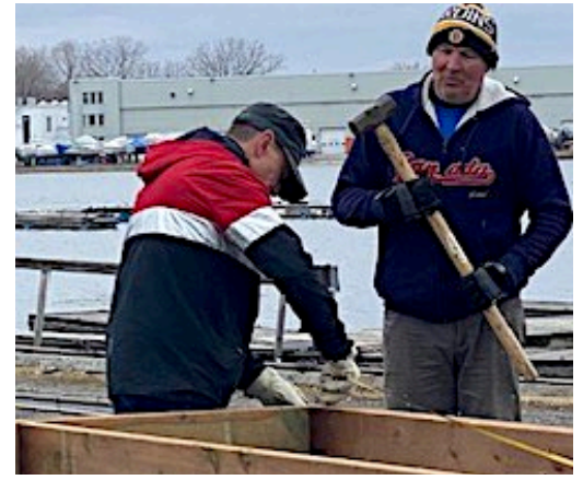
Mike Simic prepares to use the 'Monday hammer' to square up a dock frame prior to the deck boards going on. This dock was successfully squared to within \frac{1}{8} of an inch over its 32 ft. length.
