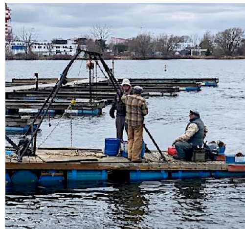
Raising a dock with the barge crane winch in order to check the anchors.
