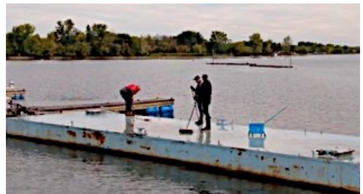
Preparing the blue dock for a coat of paint during Oct.1 work party.
