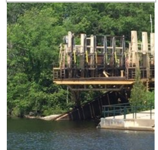
Big Chute marine railway at Lock 44 carries boats in individual cradles over 60 ft. height change.
