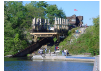
Big Chute marine railway at Lock 44 carries boats in individual cradles over 60 ft. height change.
