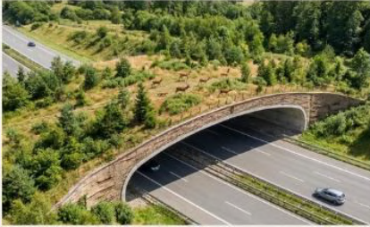
Eco bridge / wildlife overpass
