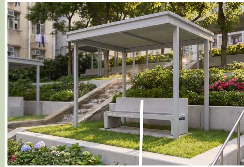
pavilion-like structure for shading
